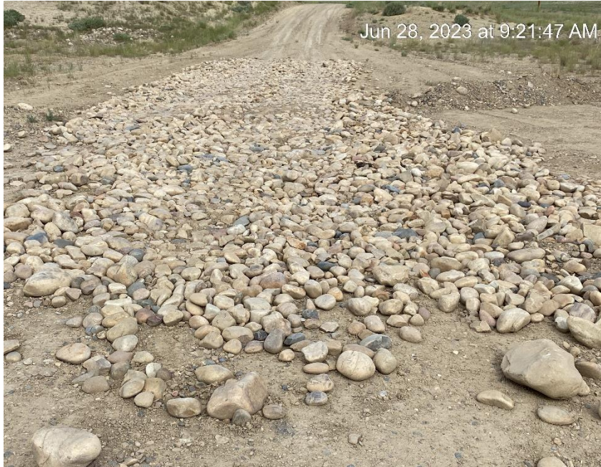
West entrance tracking pad installed since last inspection
