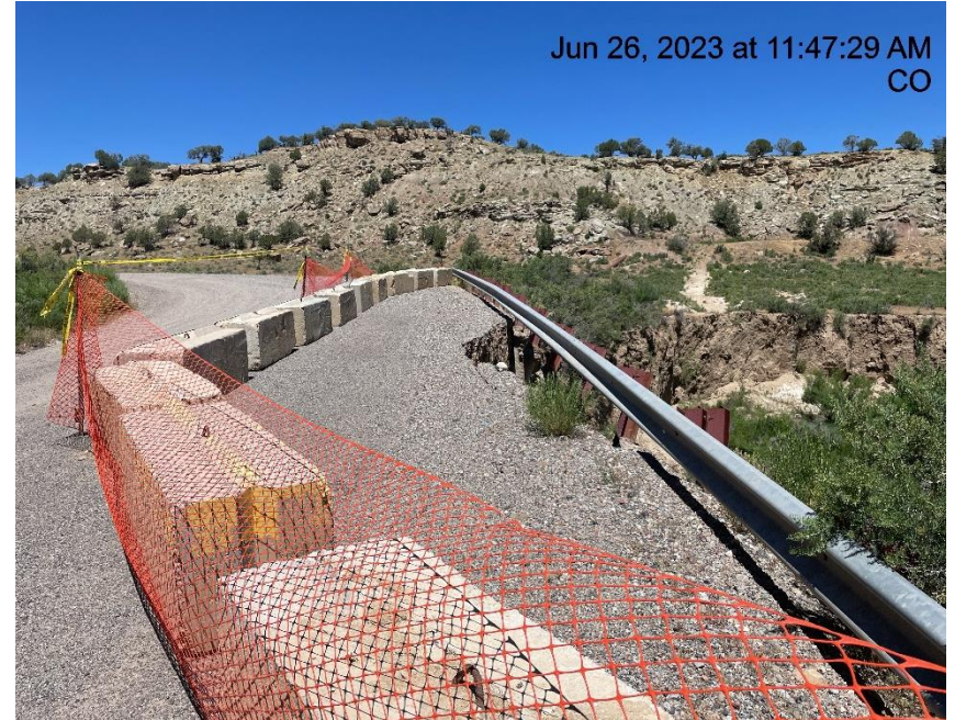
Photo # 1924 Damaged section of access road
