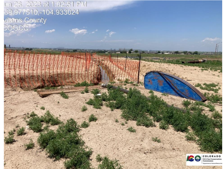
Pic 2 stormwater issue on location, horses head needs to be removed.
