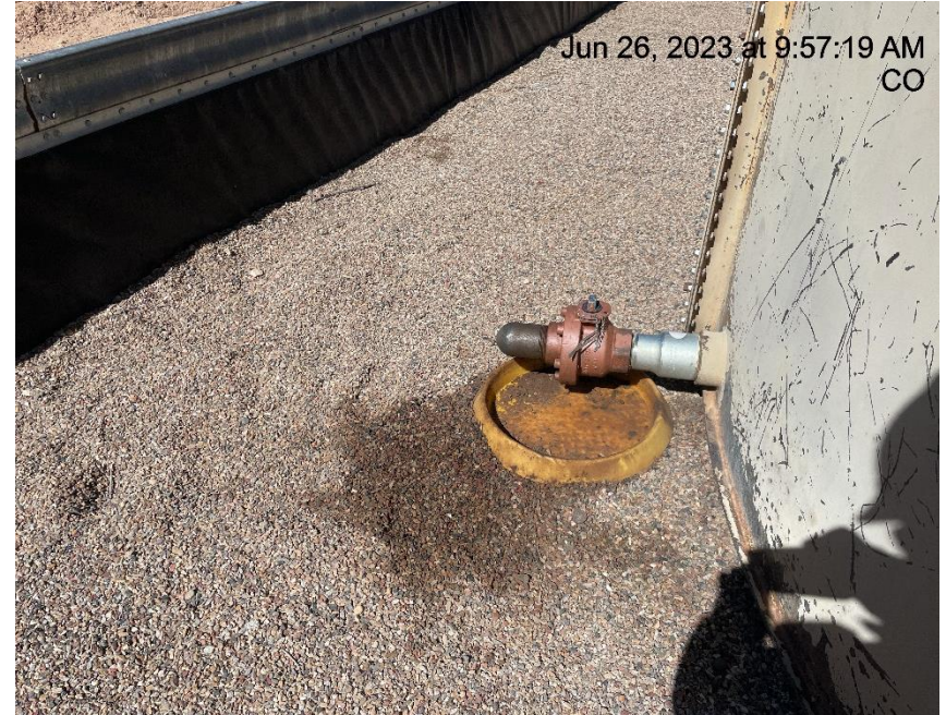
Photo # 1798 Stained gravel in secondary containment
