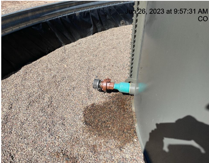
Photo # 1799 Stained gravel in secondary containment
