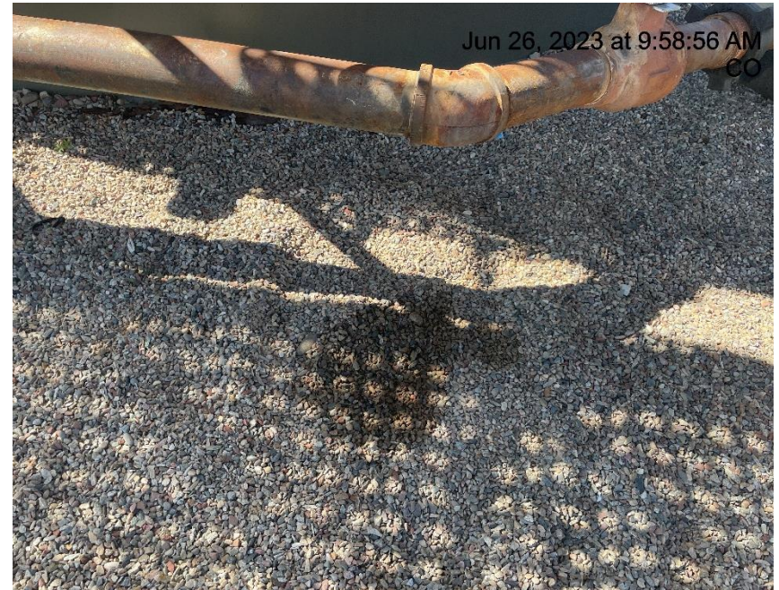
Photo # 1800 Stained gravel in secondary containment
