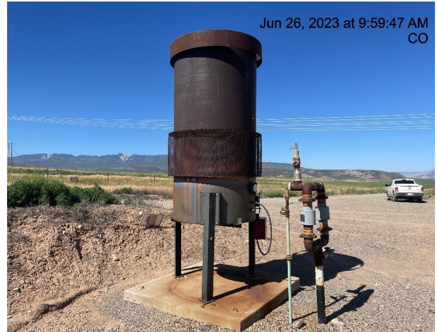
Photo # 1802 Unused equipment/ECD is completely disconnected
