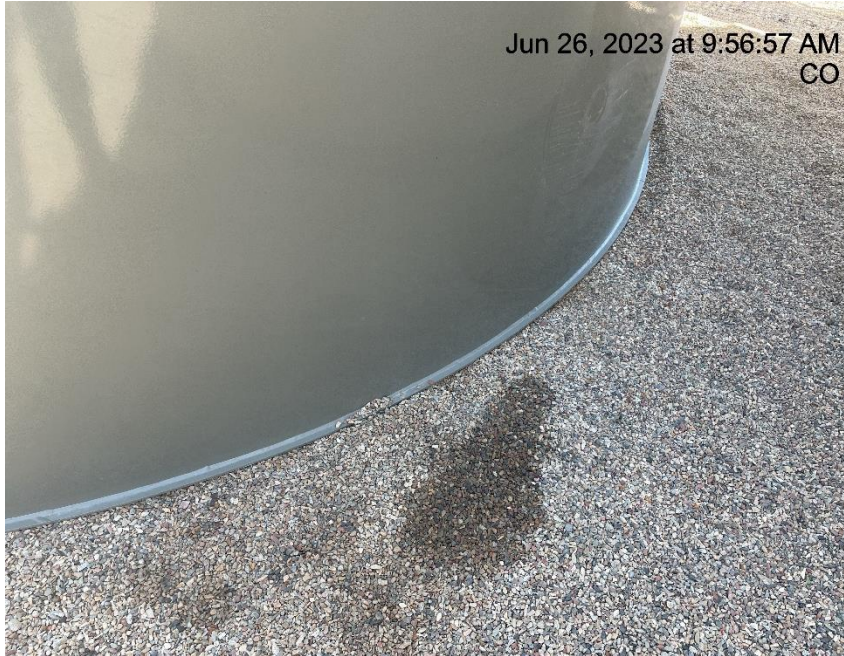
Photo # 1797 Stained gravel in secondary containment
