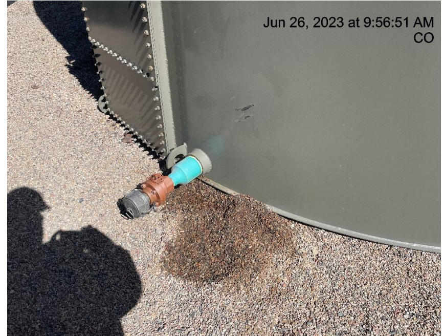
Photo # 1796 Stained gravel in secondary containment
