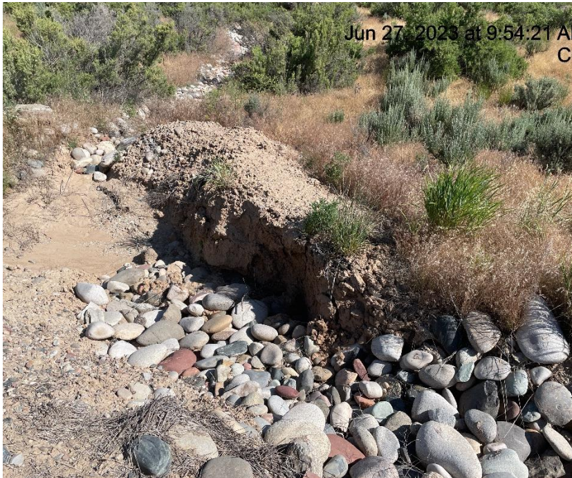
Photo # 1987 Sediment trap needs maintenance
