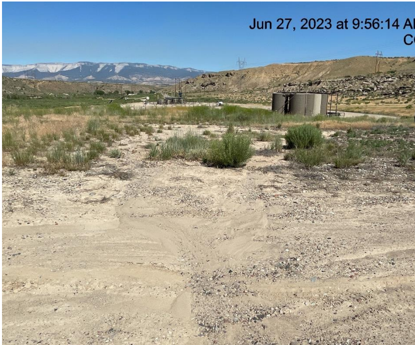
Photo # 1992 Erosion & transport of sediment off location/sediment chocking of vegetation
