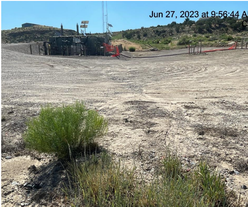
Photo # 1994 Erosion & transport of sediment off location/sediment choking of vegetation
