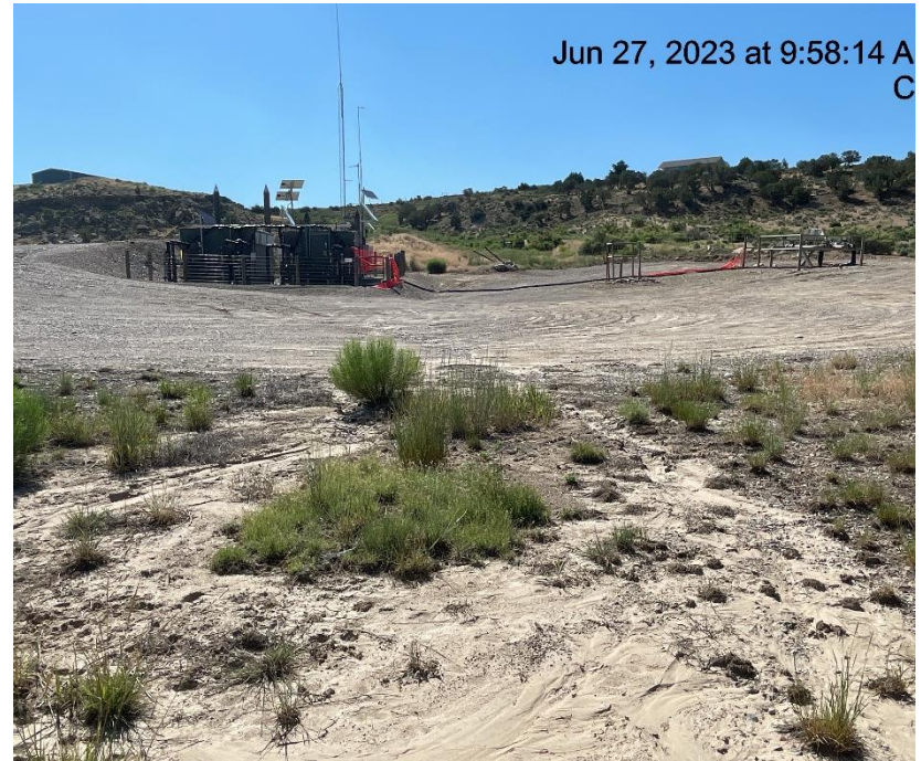
Photo # 2002 Erosion & transport of sediment off location/sediment choking of vegetation
