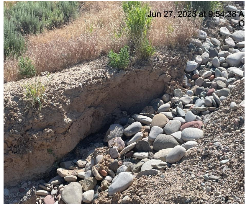
Photo # 1988 Sediment trap needs maintenance
