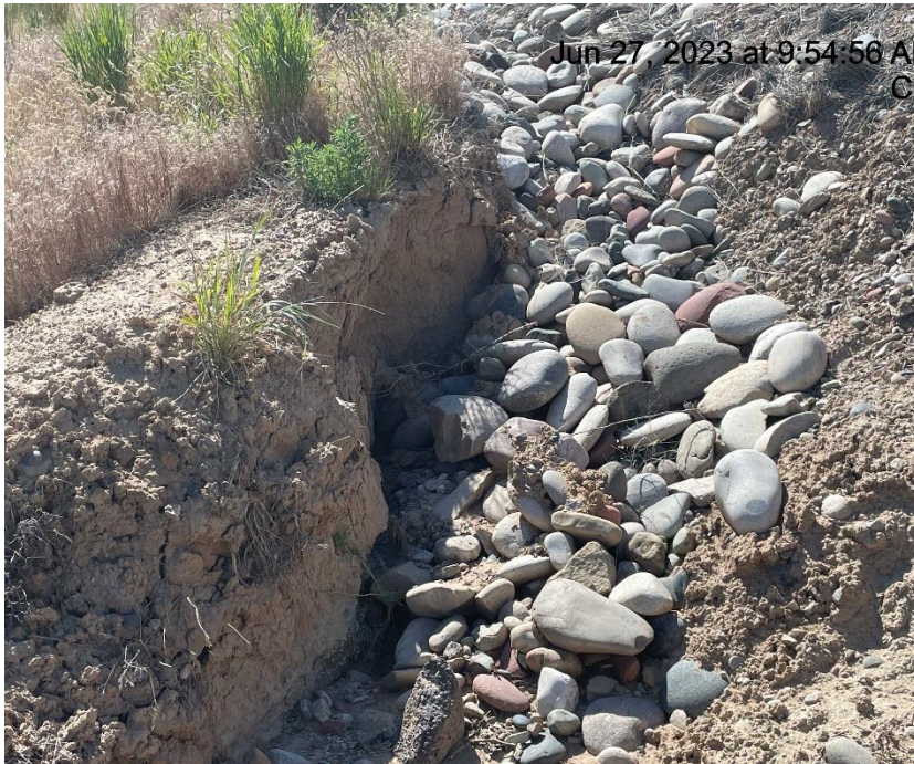
Photo # 1989 Sediment trap needs maintenance
