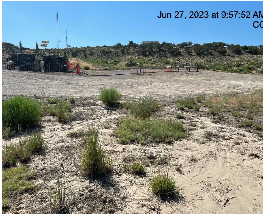
Photo # 1999 Erosion & transport of sediment off location/sediment choking of vegetation
