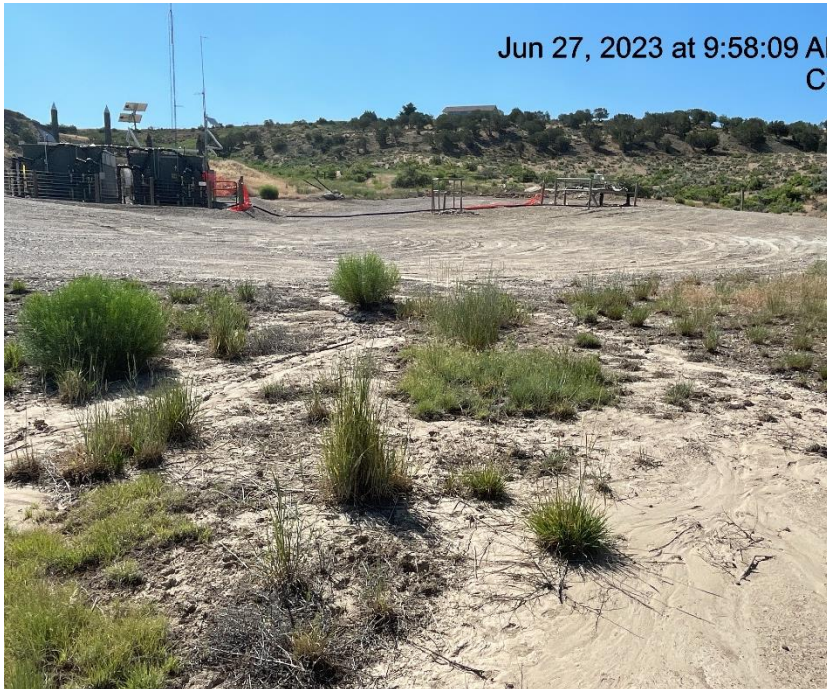
Photo # 2001 Erosion & transport of sediment off location/sediment choking of vegetation
