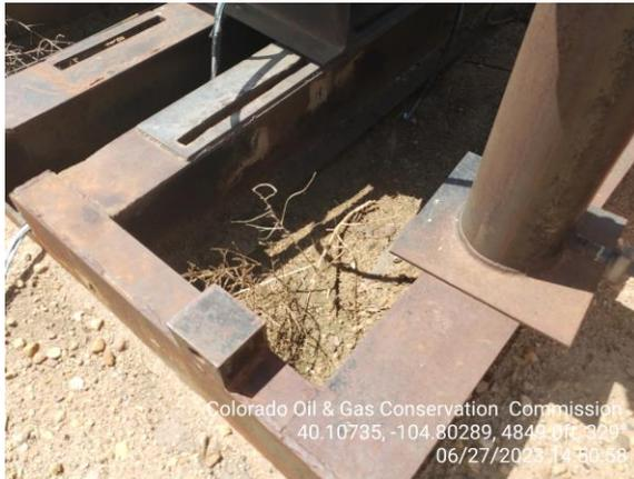
**Photo 13 stained soil in the pump jack frame.**
