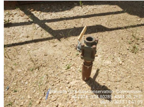
**Photo 5 Unused Flow line with valve next to pump jack no LOTO.**
