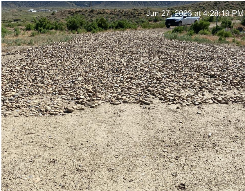
Tracking pad installed since last inspection
