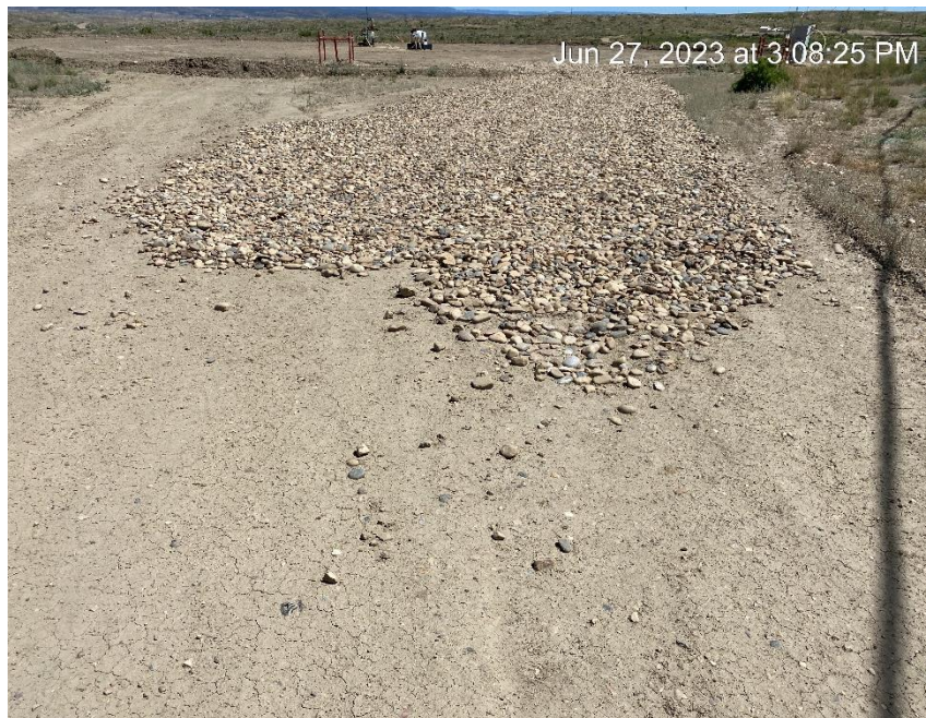
Tracking pad installed since last inspection
