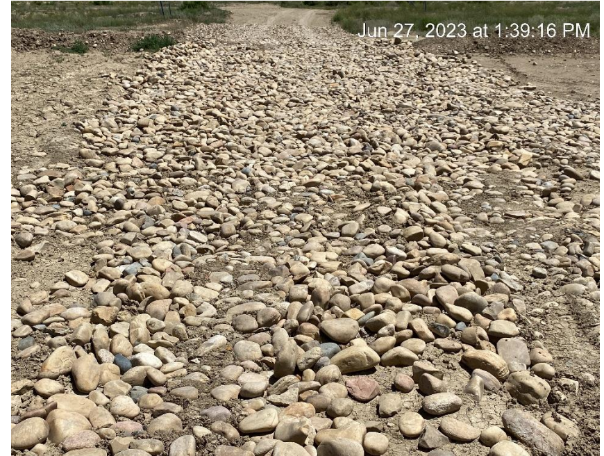
East entrance tracking pad installed since last inspection
