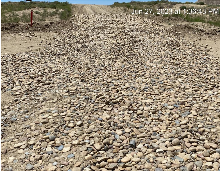
Northwest entrance tracking pad installed since last inspection
