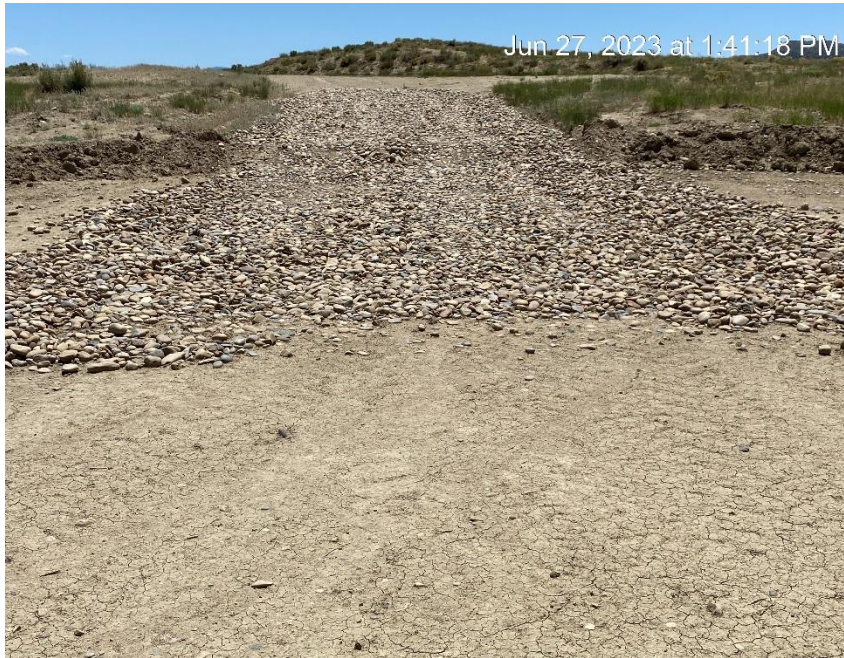
South entrance tracking pad installed since last inspection
