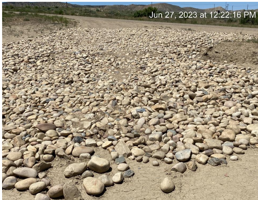
Vehicle tracking pad installed since last inspection
