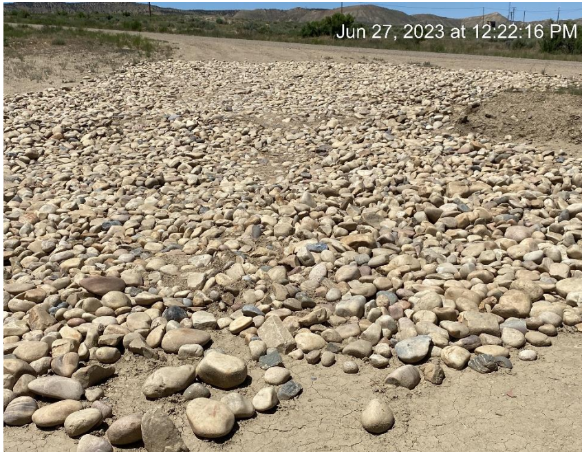
Vehicle tracking pad installed since last inspection
