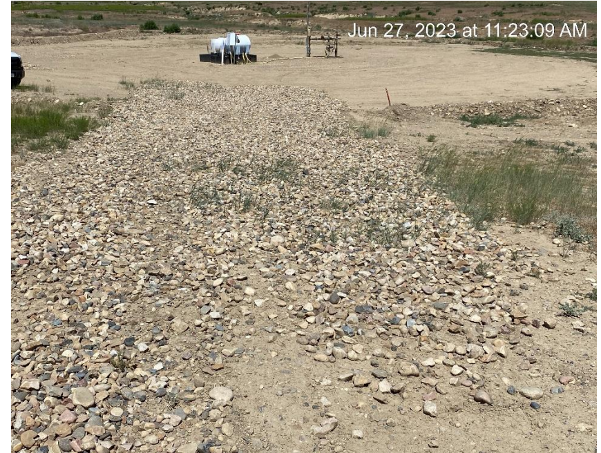
Vehicle tracking pad installed since last inspection
