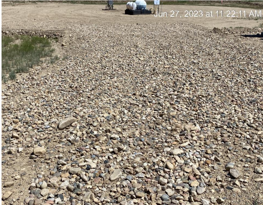
Vehicle tracking pad installed since last inspection
