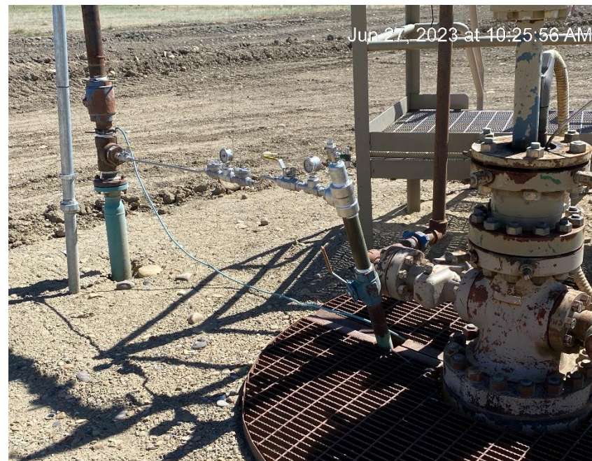
Surface casing plumbed into flowline
