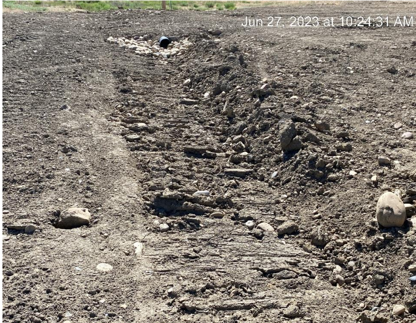
Sediment trap added since last inspection
