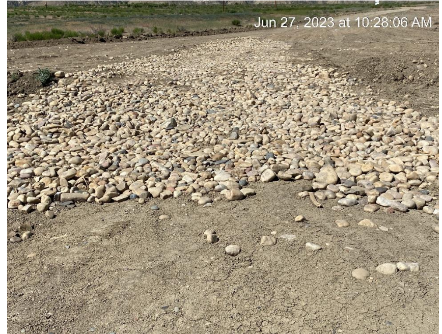
Vehicle tracking pad added since last inspection
