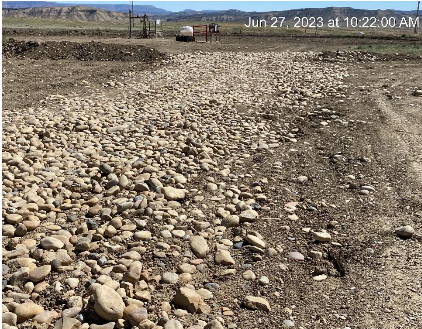
Vehicle tracking pad added since last inspection
