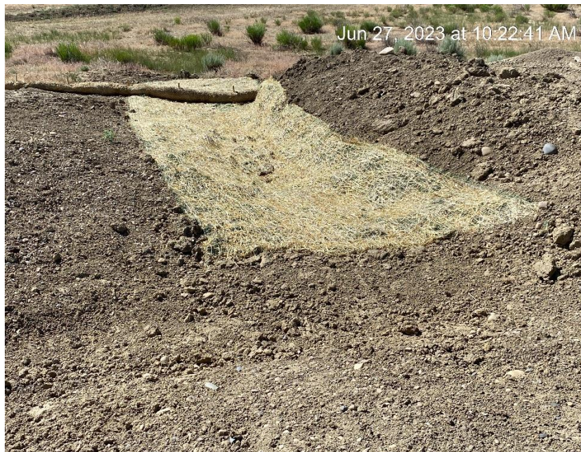
Drainage repaired since last inspection
