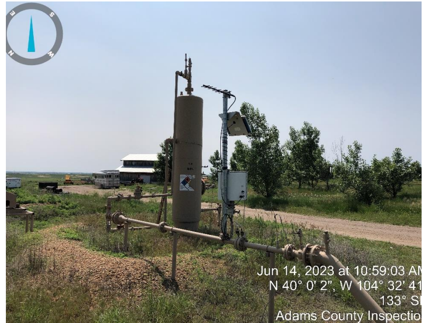
Photo# 2 Meter & separator
