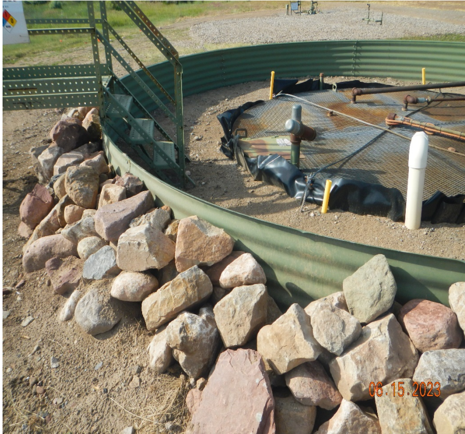
Photo 4. The secondary containment has been reinstalled into the ground. Larger rock rip/rap has been placed around the containment.
