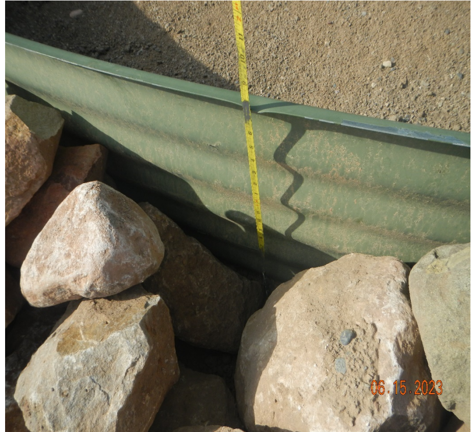
Photo 5. The lowest point of the containment sits approximately 1ft. 8 inches above ground level.
