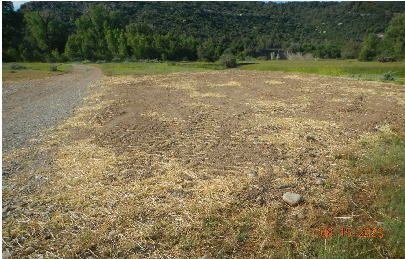
Photo 7. Facing toward the southwest side of the location. This area has been regraded and seeded. Most of the mulch has blown off and soils are not stabilized.
