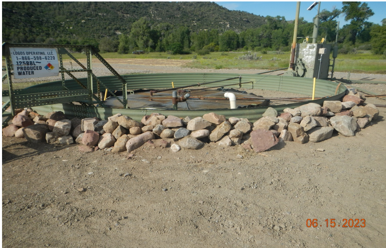
Photo 3. Facing toward the open top tank. The secondary containment has been reinstalled into the ground. Larger rock rip/rap has been placed around the containment.
