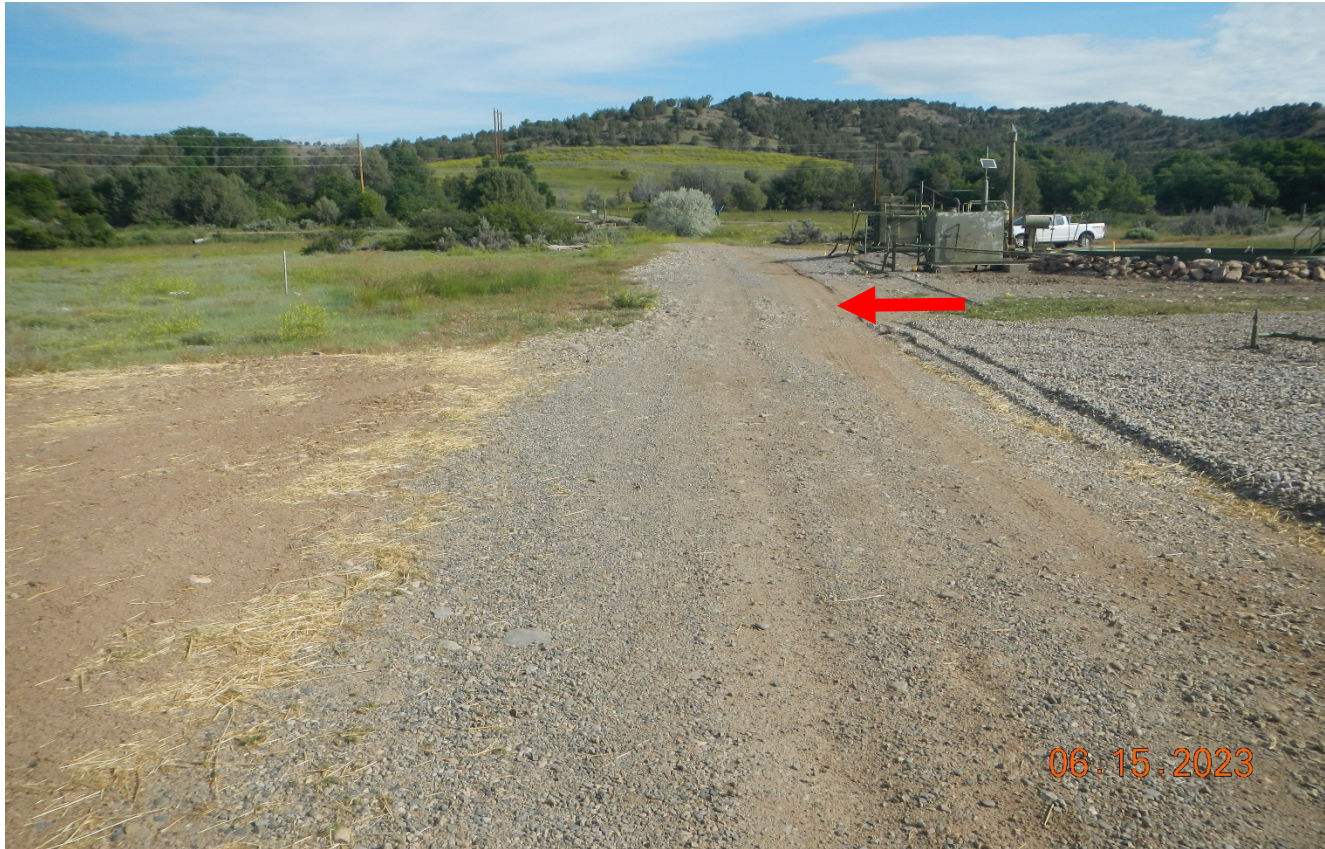
Photo 9. Facing north toward the location. The area of the road shows signs of scouring where flood flowed across the road from right to left towards the Florida River.
