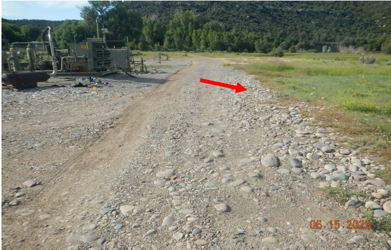
Photo 10. Facing south toward the location. The area of the road shows signs of scouring where flood flows across the road from left to right towards the Florida River. No BMPs have been installed in this area.
