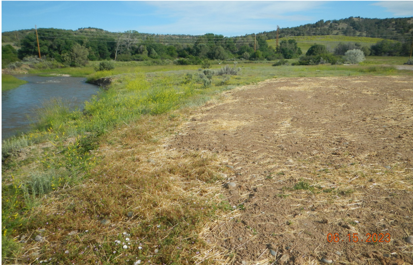
Photo 8. Facing north along the the Florida River. There is no stormwater controls installed along the disturbed soils adjacent to the river which is a concern.
