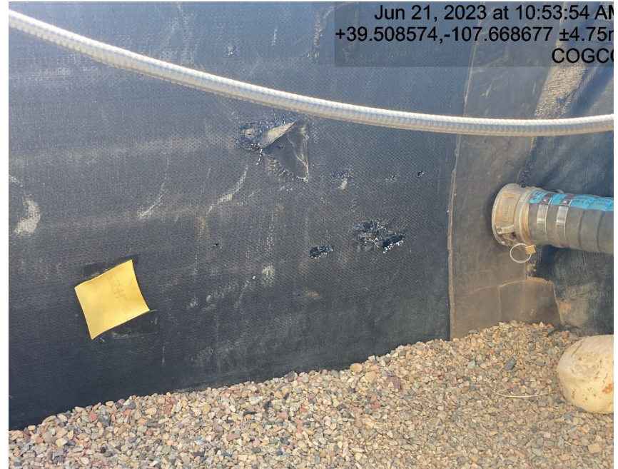
Holes in containment
