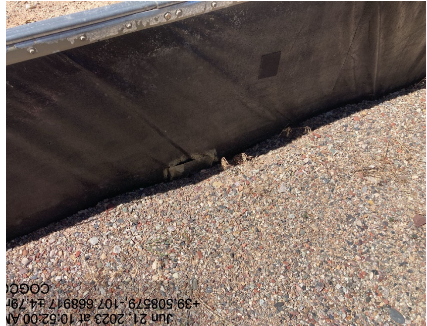
Holes in containment
