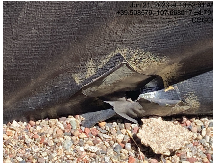
Holes in containment
