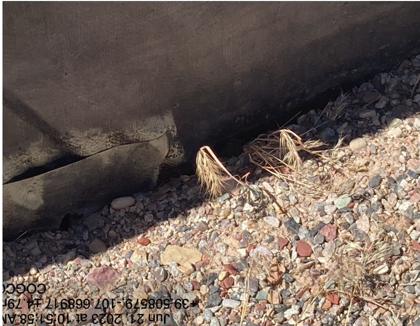
Holes in containment
