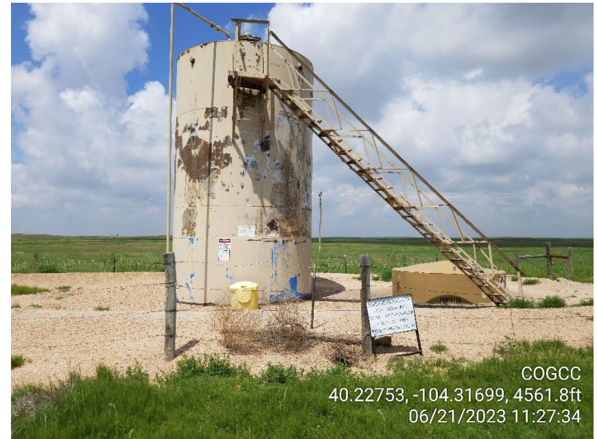
Photo 2 – Tank Battery
