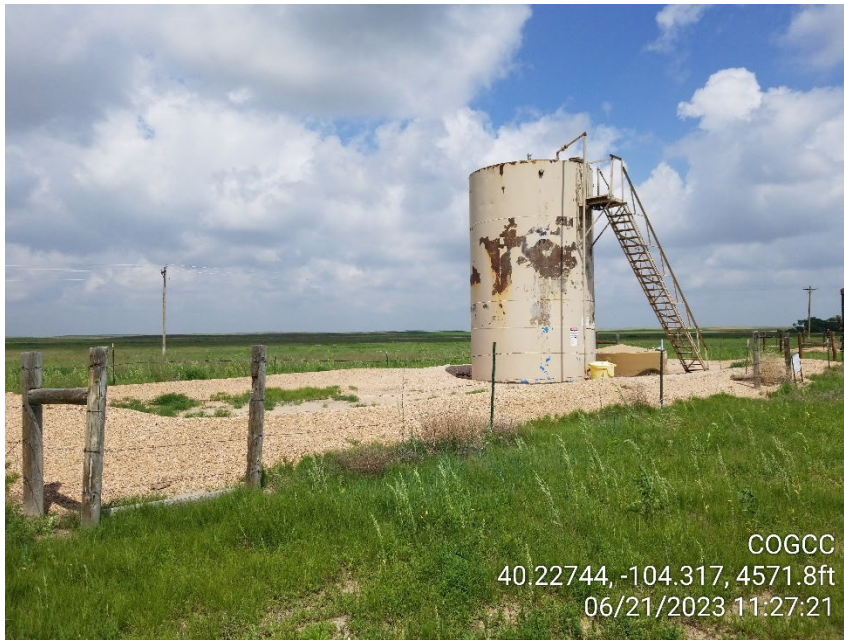
Photo 1 – Tank Battery – Weeds in Berm
