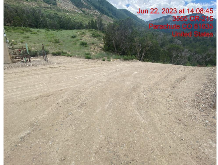
Insufficient Vehicle Tracking BMPs at Location Entrance/Exit – Photo #04720
