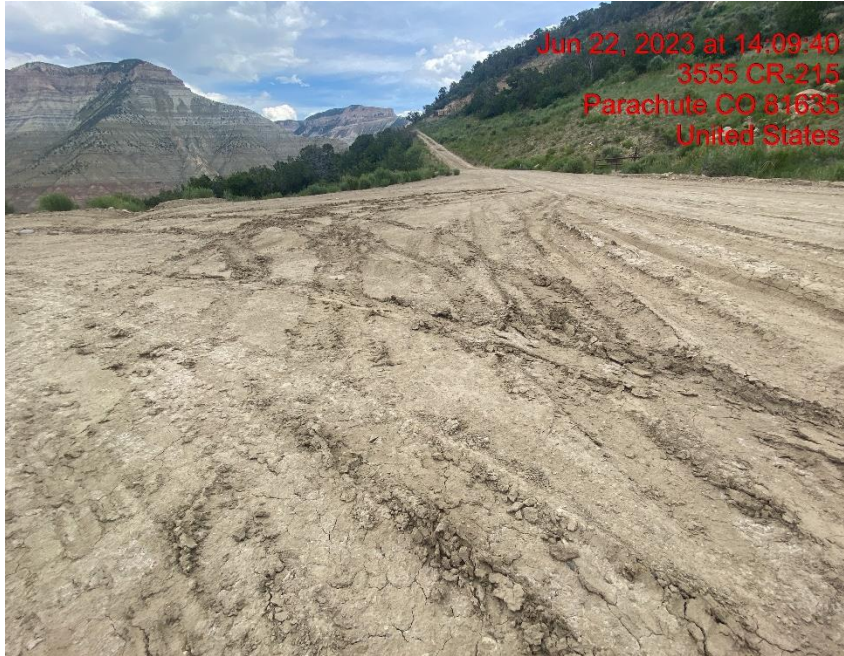
Location Lacks Stabilization – Photo #04722
