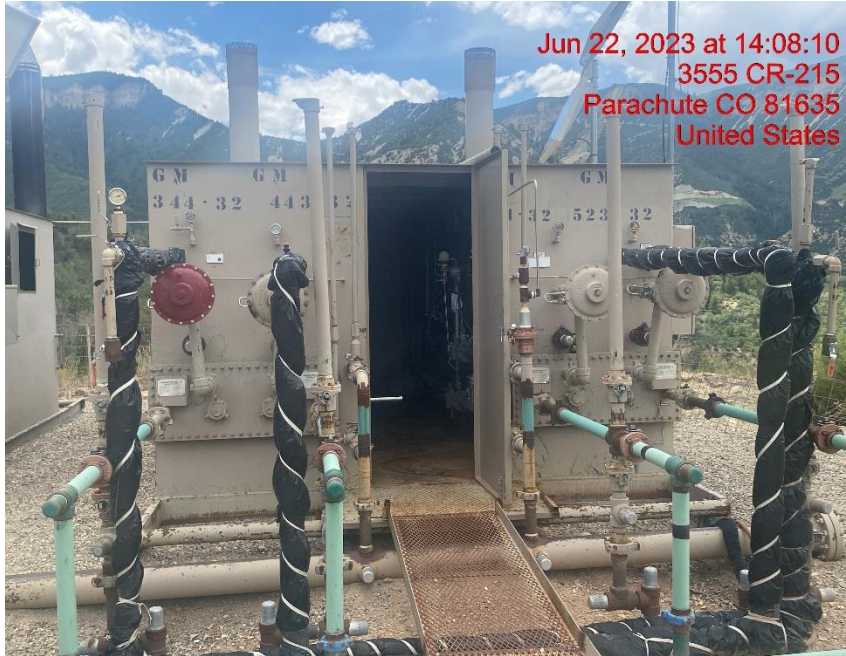
Unsecured Door on Separator – Photo #04718
