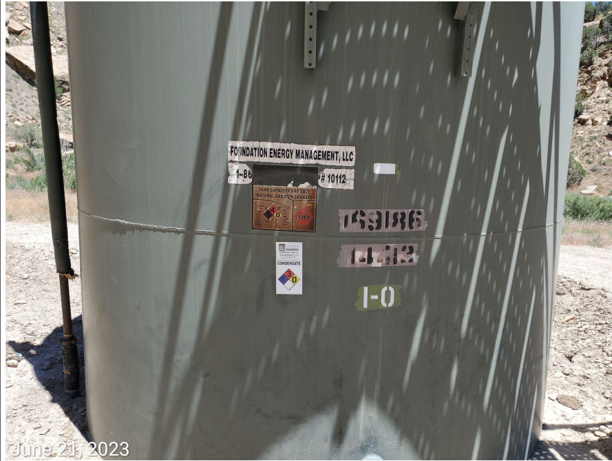
Photo 2: Signage/labels at the condensate and produced water tanks remain out of compliance with 605 rules.
