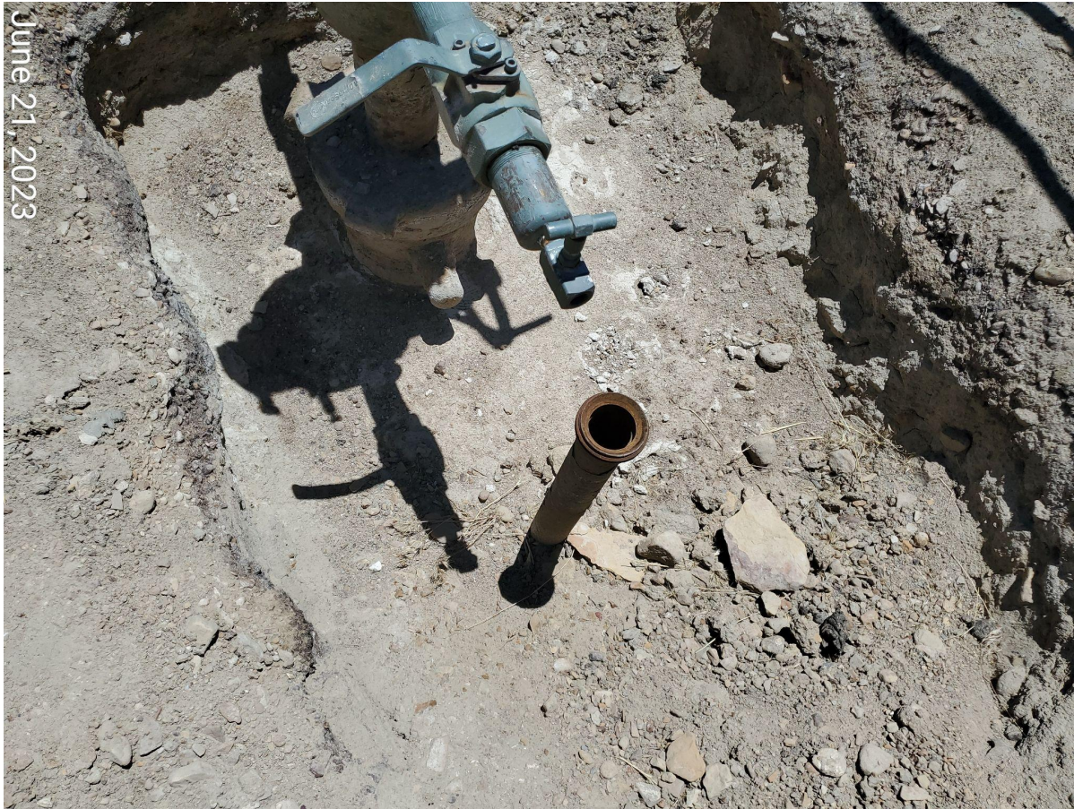
Photo 4: Photo taken from the wellhead. Photo shows Operator has removed sections of the pipe from the well, leaving an open/exposed riser pipe.
