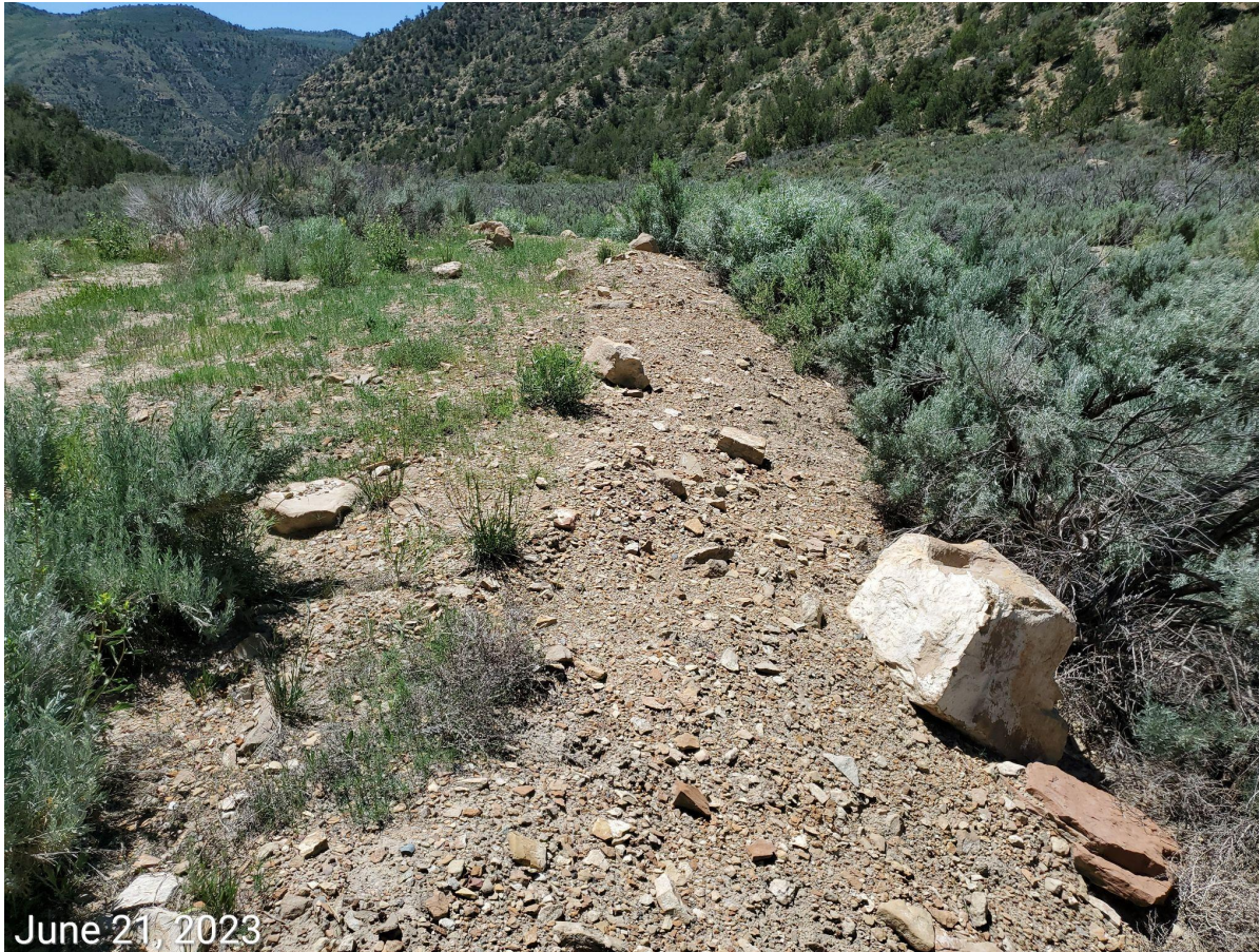
Photo 8: Fill slopes. Location requires compaction alleviation, recontouring/regrading and reclamation.
