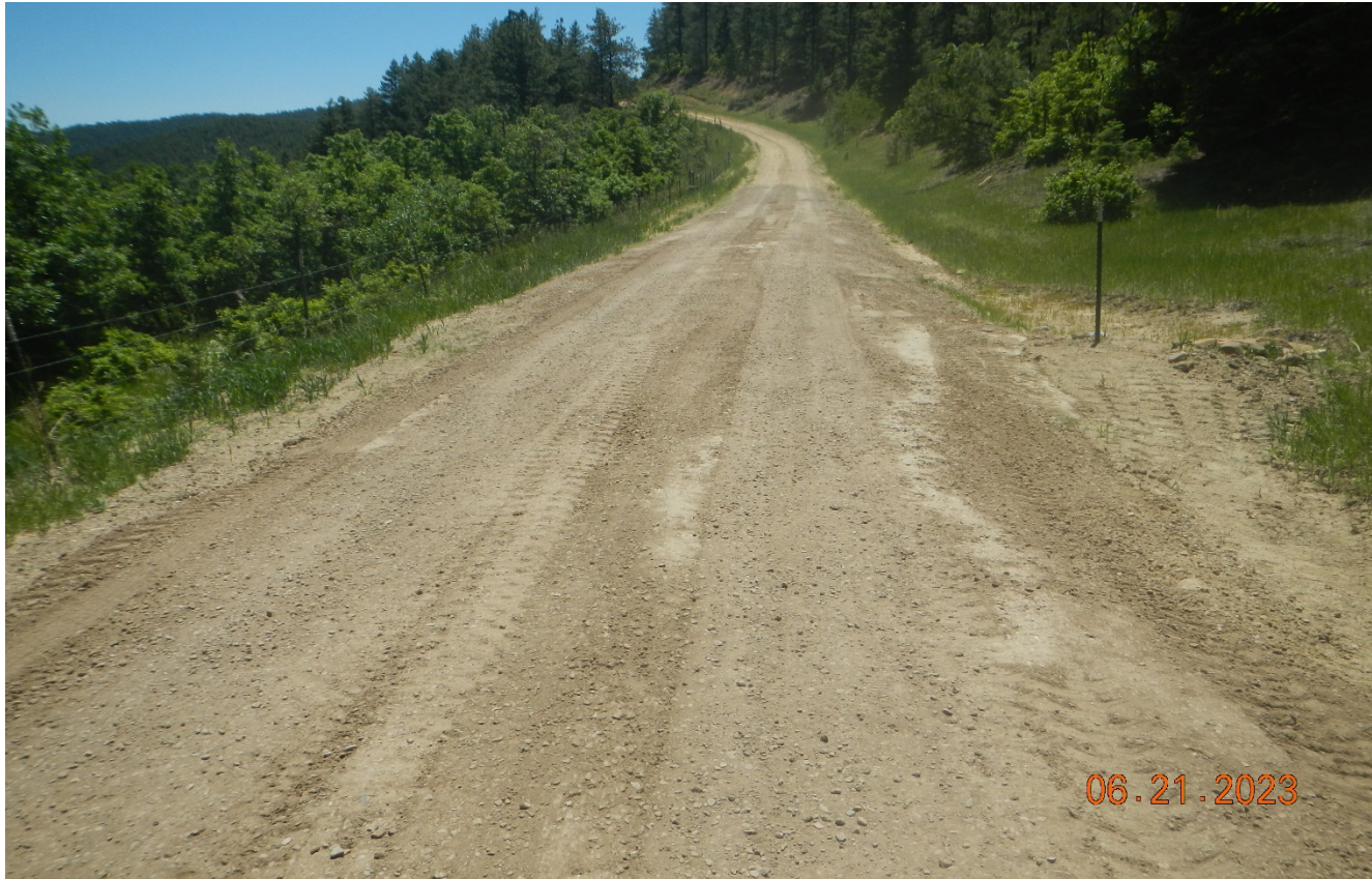
Photo 2. Facing southeast along the road. There has been road base applied to this area of the road where stormwater use to accumulate and culvert is maintained.
