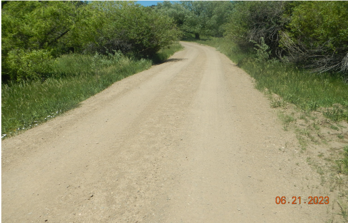
Photo 1. Facing west along the main road in Jaroso Canyon. There has been road base applied to this area of the road where stormwater use to accumulate.
