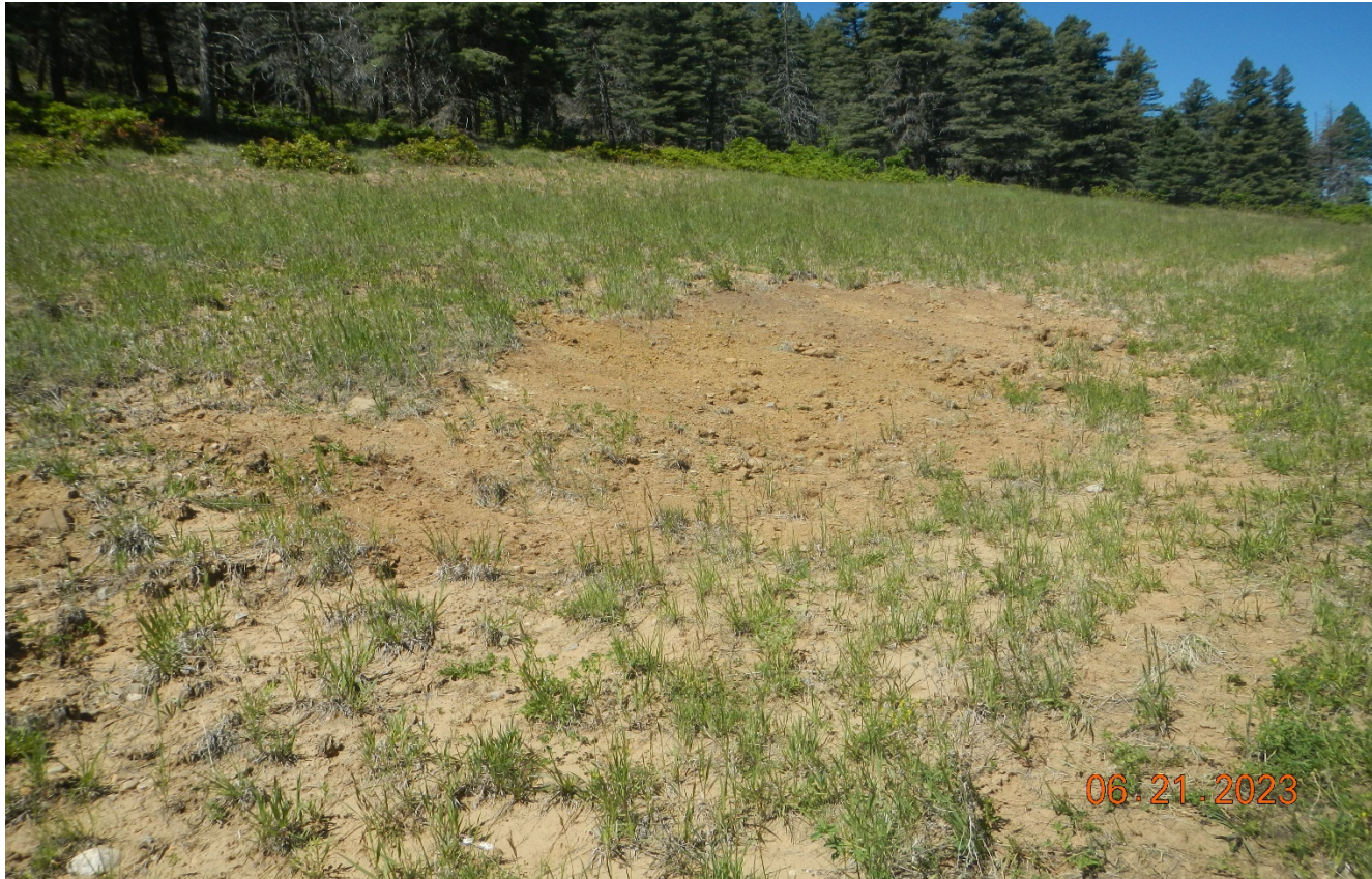
Photo 1. Facing west at the location. The area of erosion has been repaired and seeded. Vegetation will need to establish for long term stabilization.
