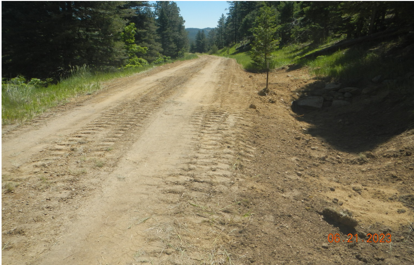
Photo 2. Facing east along the pre-existing access road. This culvert has been cleaned out. The disturbance areas have been seeded and vegetation will need to reestablish.
