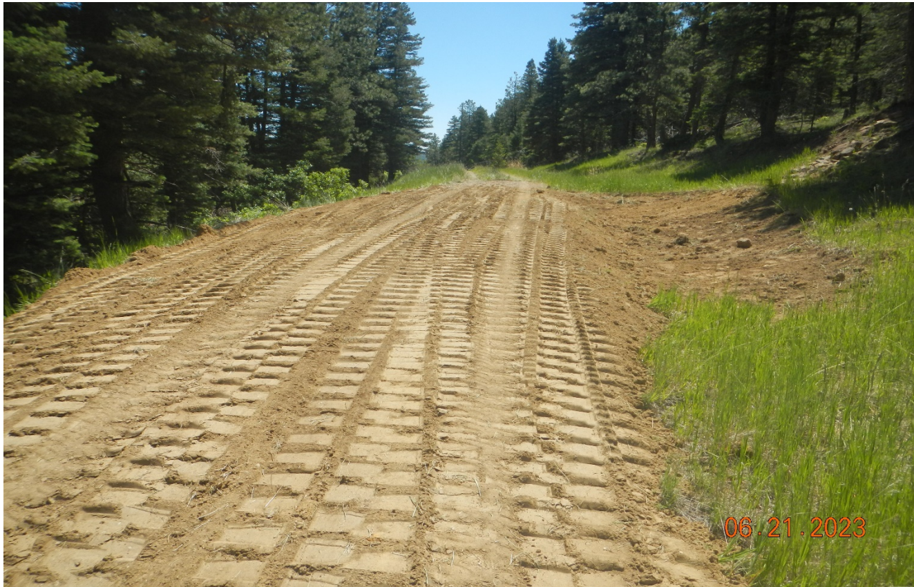
Photo 1. Facing east along the pre-existing access road. This culvert has been cleaned out. The disturbance areas have been seeded and vegetation will need to reestablish.
