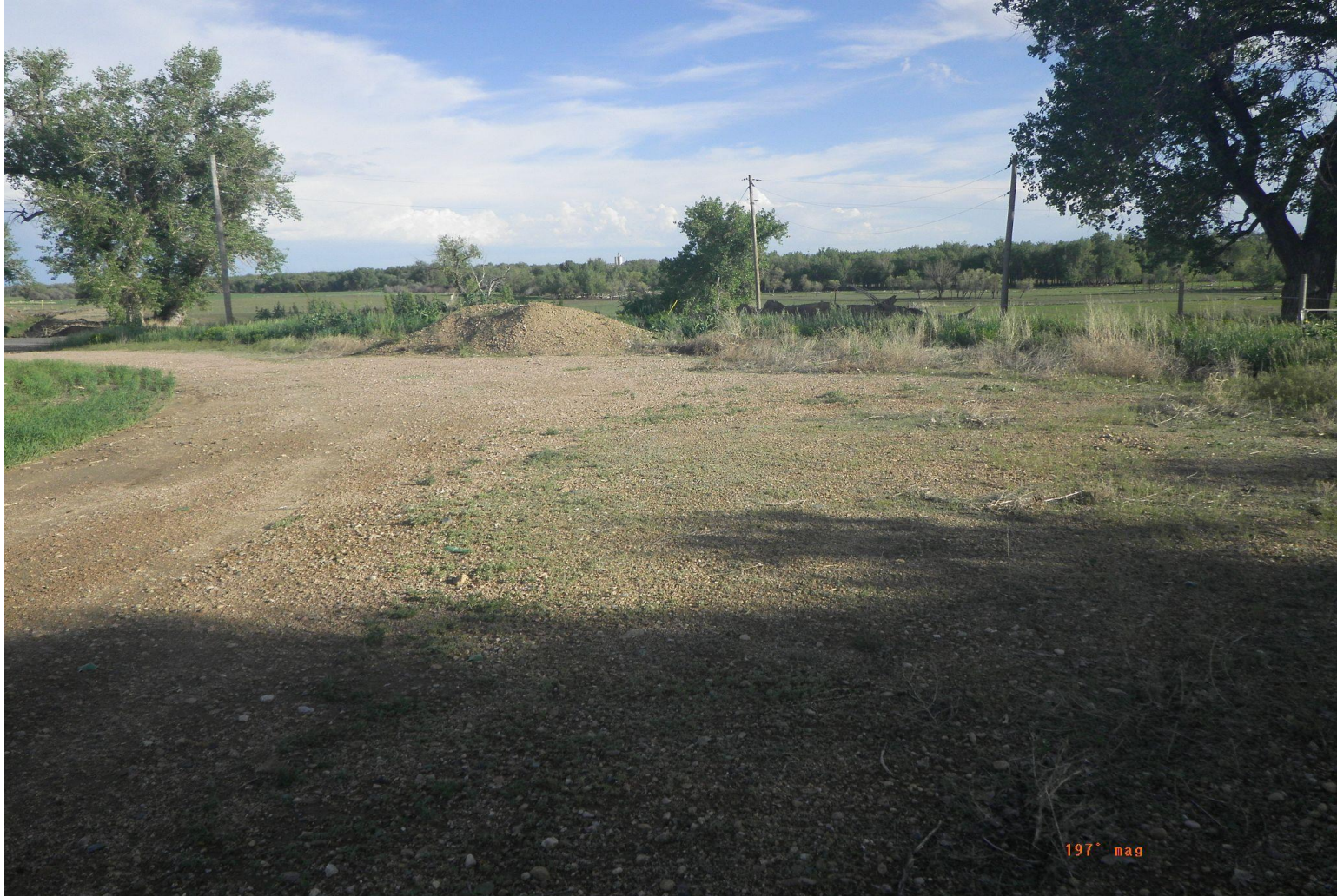
Photo 6. Overview photo of the tank battery taken at ground level from the northern edge facing south.
