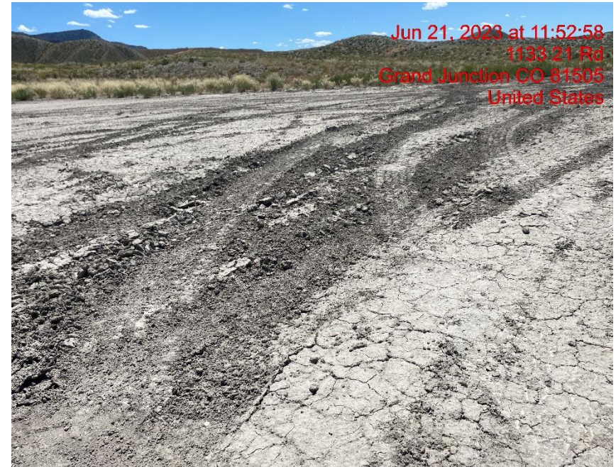
Location Lacks Stabilization – Photo #04644
