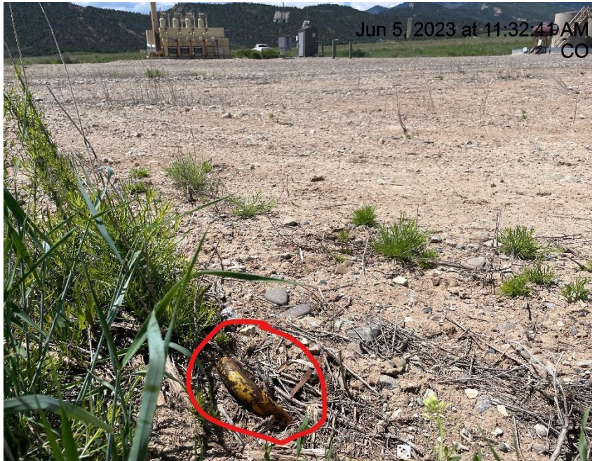
Photo # 9521 From Inspection 708900689 conducted on 06/05/2023 Unmarked deadman
