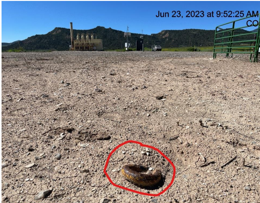
Photo # 1553 Unmarked deadman from a different angle
