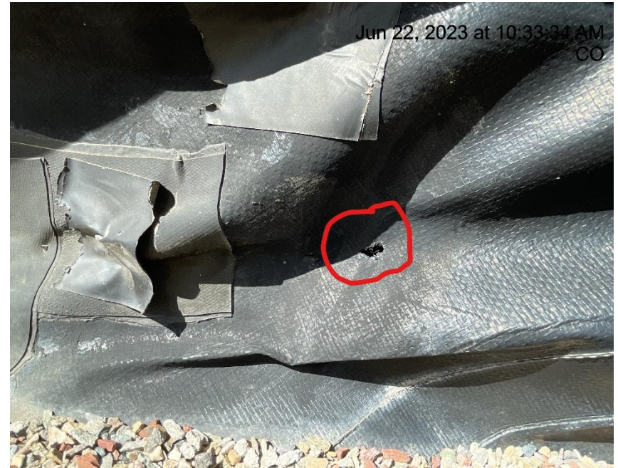
Photo # 1461 Hole in secondary containment liner/liner needs maintenance
