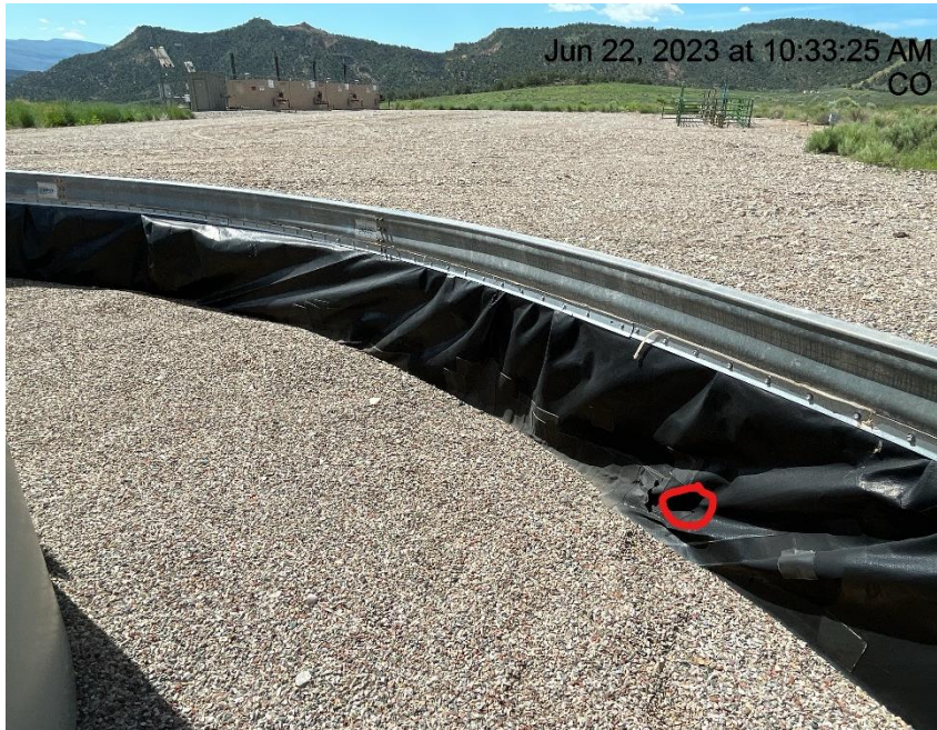
Photo # 1460 Hole in secondary containment liner/liner needs maintenance
