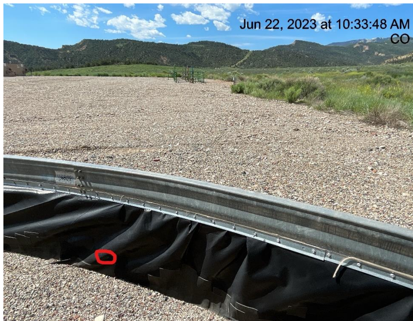
Photo # 1463 Hole in secondary containment liner/liner needs maintenance
