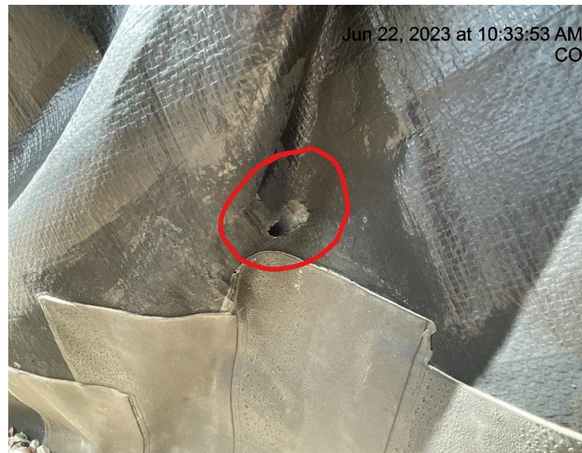
Photo # 1464 Hole in secondary containment liner/liner needs maintenance
