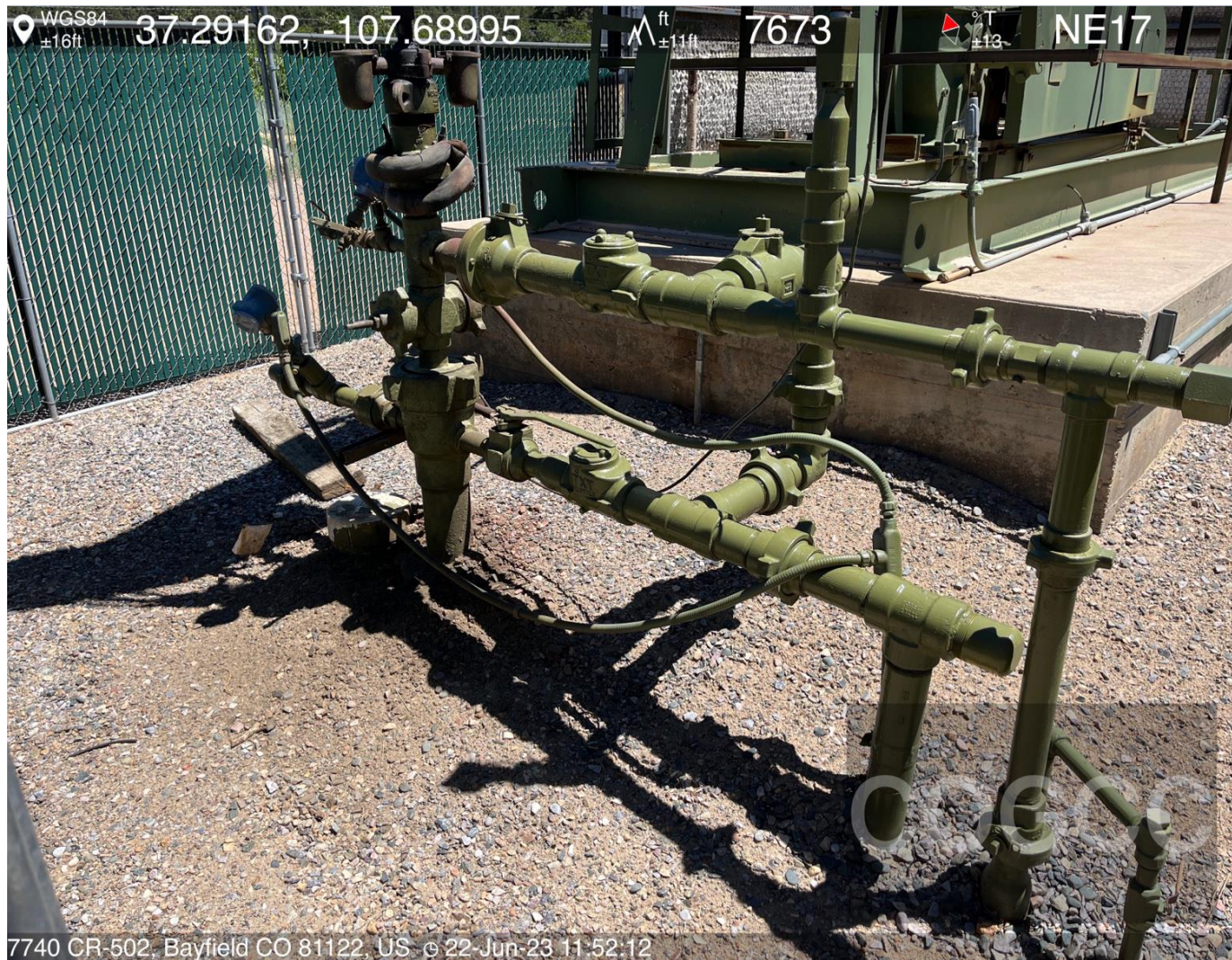
Photo #2 View of the wellhead assembly.
