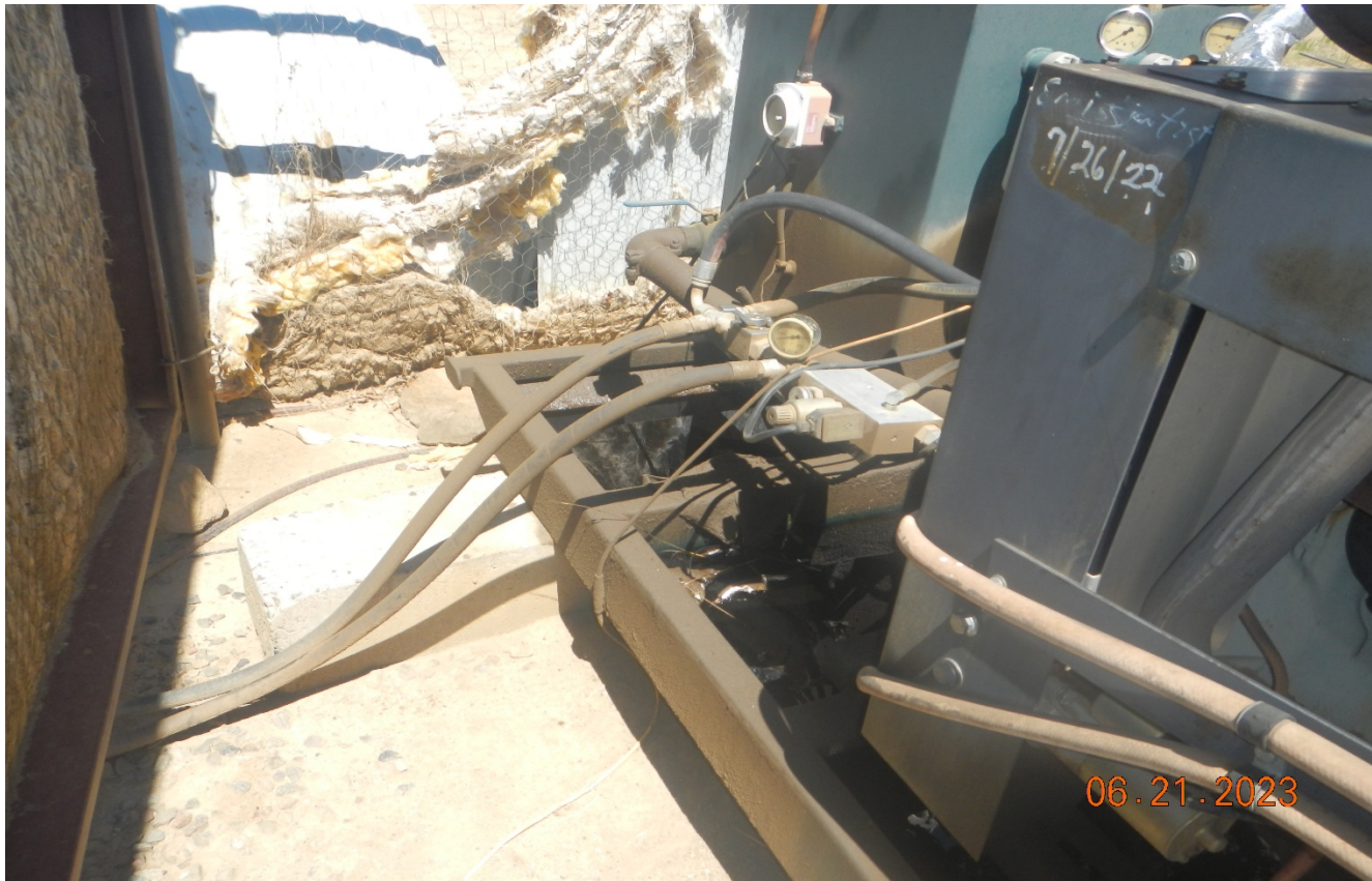
Photo 2. There is oily fluids inside the engine skid that need to be cleaned up.
