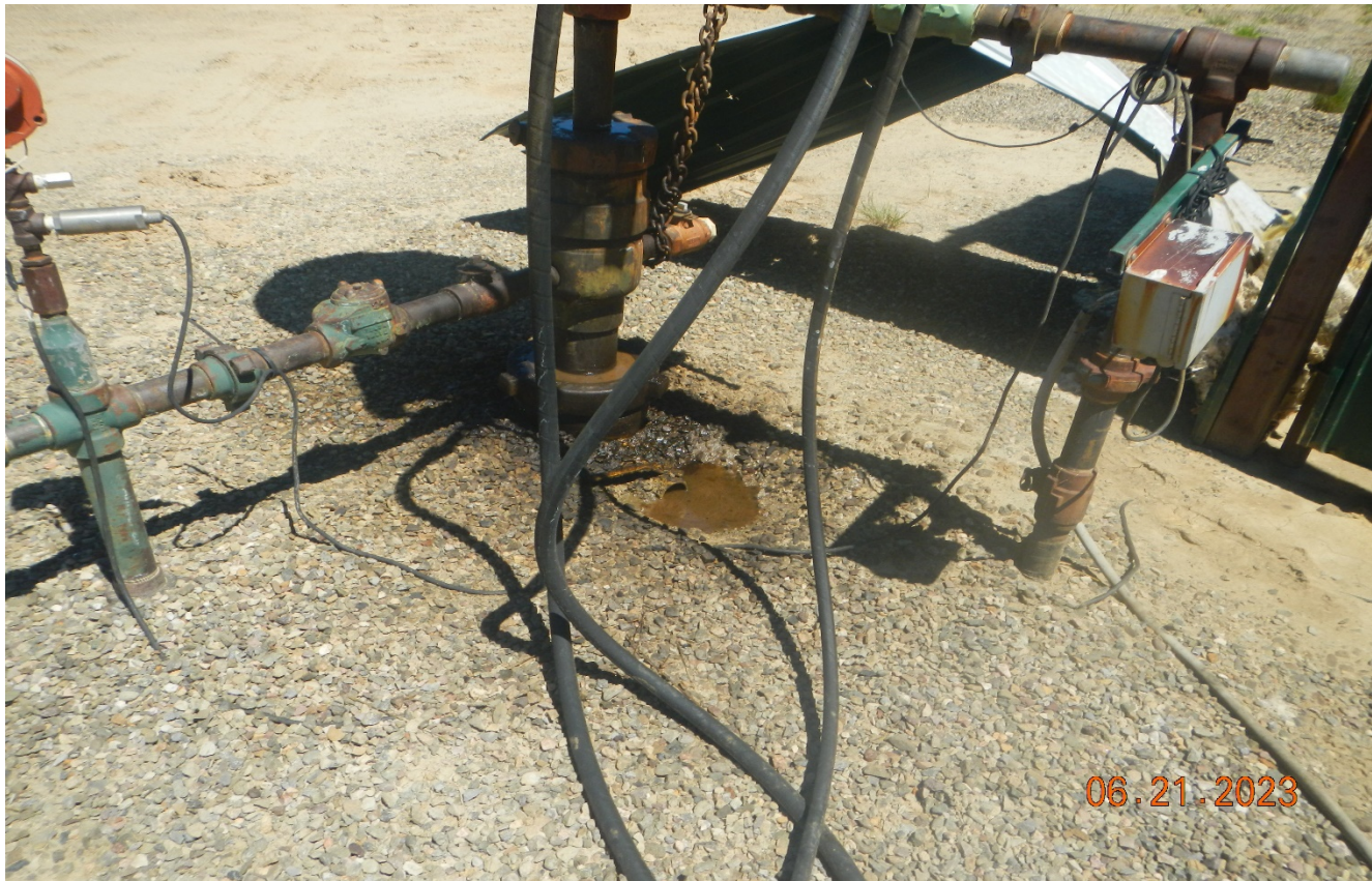
Photo 3. There is a oily fluids at the wellhhead that need to be cleaned up.
