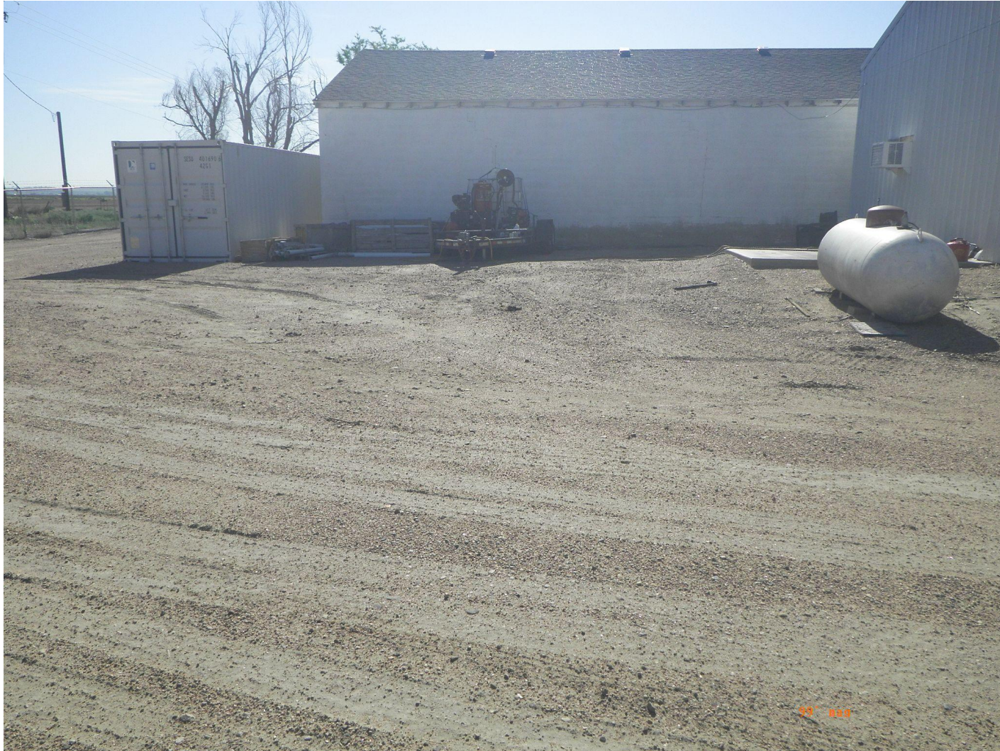
Photo 5. Overview photo of the tank battery. Note: tank battery falls within a storage area of ARB Midstream company.
