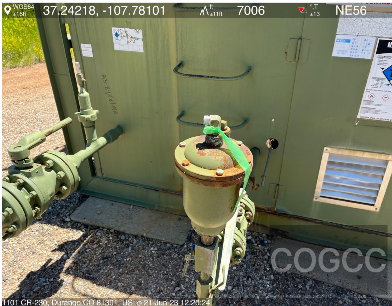
Photo #3 View of observed leaking pipe fitting.
