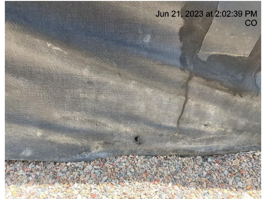
Photo # 1358 Hole in secondary containment liner/liner needs maintenance
