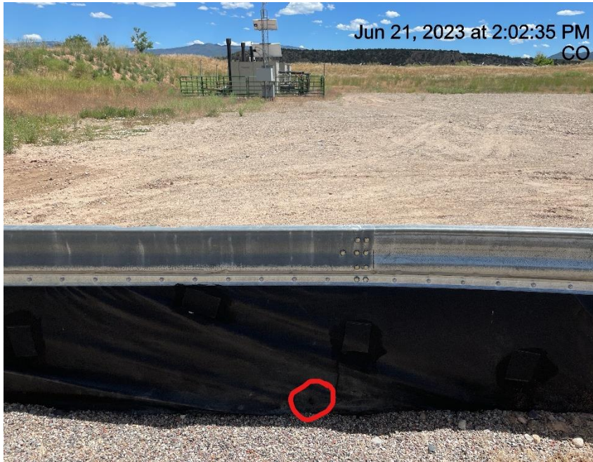
Photo # 1357 Hole in secondary containment liner/liner needs maintenance
