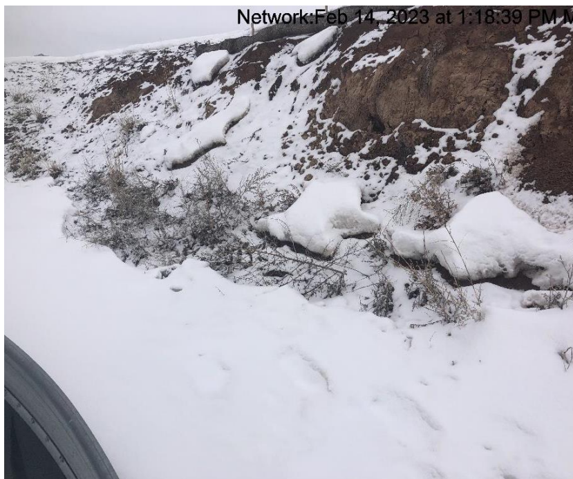
Photo # From Inspection 699805442 conducted on 02/14/2023 Slope stabilization BMP's insufficient
