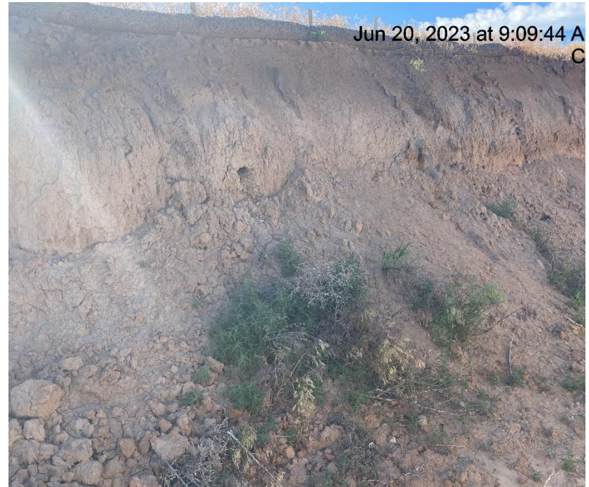
Photo # 1027 Slope stabilization BMP's insufficient
