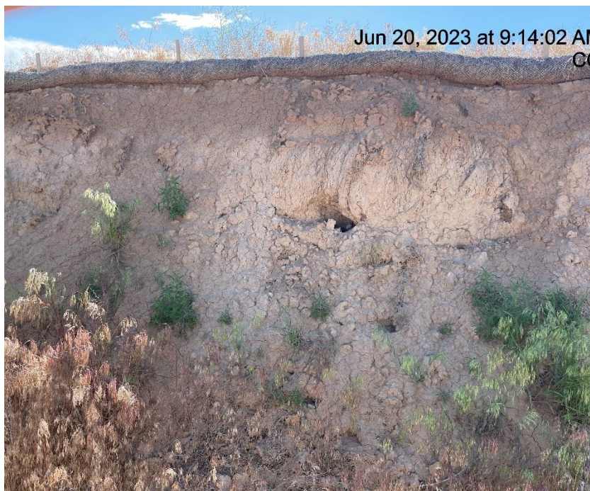
Photo # 1041 Slope stabilization BMP's insufficient
