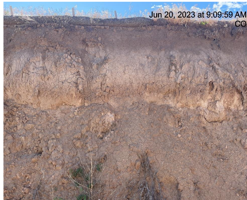
Photo # 1028 Slope stabilization BMP's insufficient
