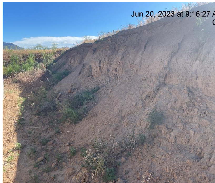
Photo # 1053 Slope stabilization BMP's insufficient
