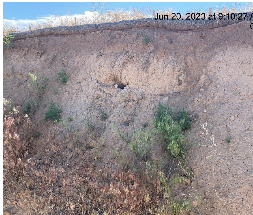
Photo # 1030 Slope stabilization BMP's insufficient
