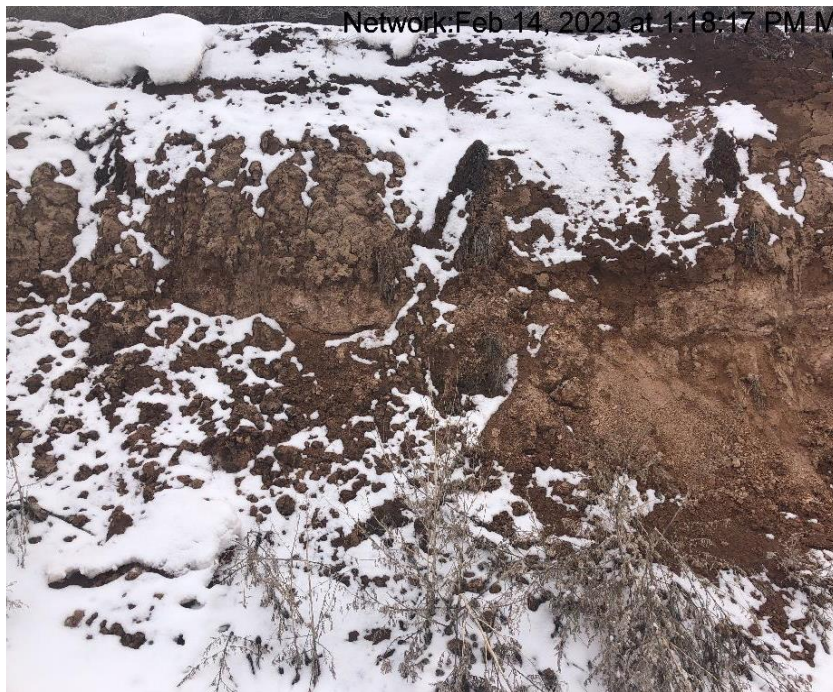
Photo # 9009 From Inspection 699805442 conducted on 02/14/2023 Slope stabilization BMP's insufficient
