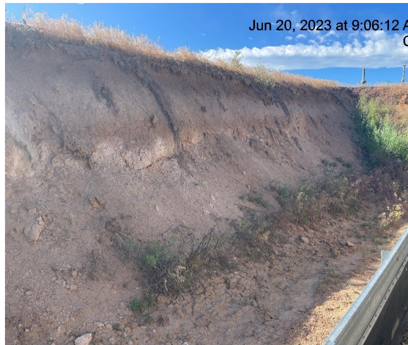
Photo # 1020 Slope stabilization BMP's insufficient
