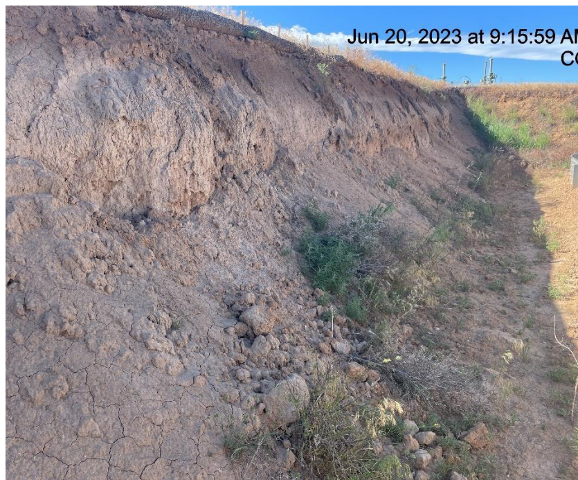
Photo # 1050 Slope stabilization BMP's insufficient
