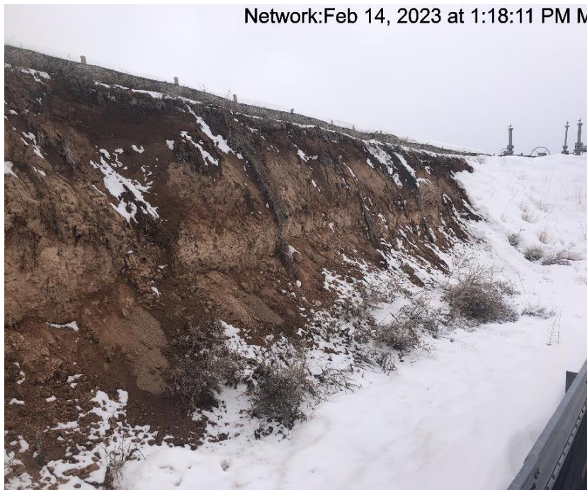
Photo # 9008 From Inspection 699805442 conducted on 02/14/2023 Slope stabilization BMP's insufficient
