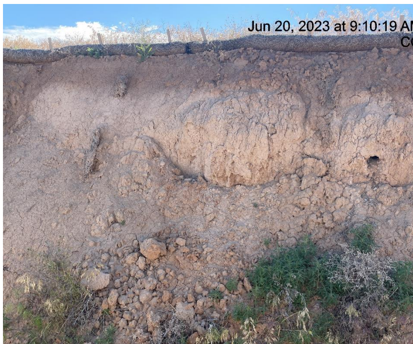
Photo # 1029 Slope stabilization BMP's insufficient
