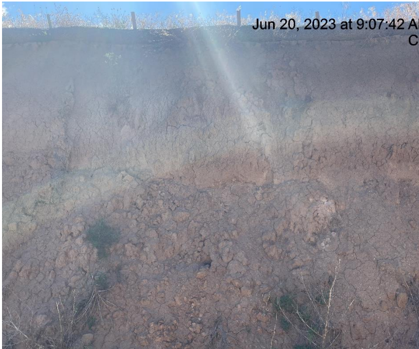
Photo # 1026 Slope stabilization BMP's insufficient
