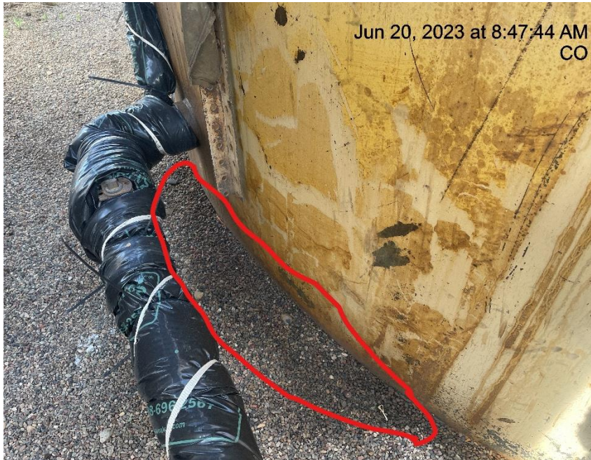
Photo # 986 Stained gravel in secondary containment
