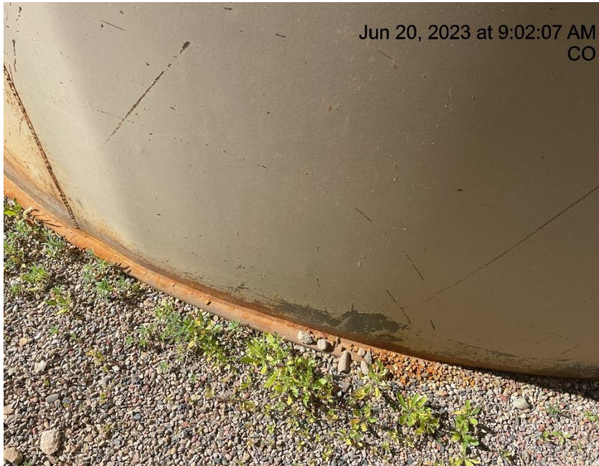
Photo # 1112 Weeds/Undesirable plant species in secondary containment
