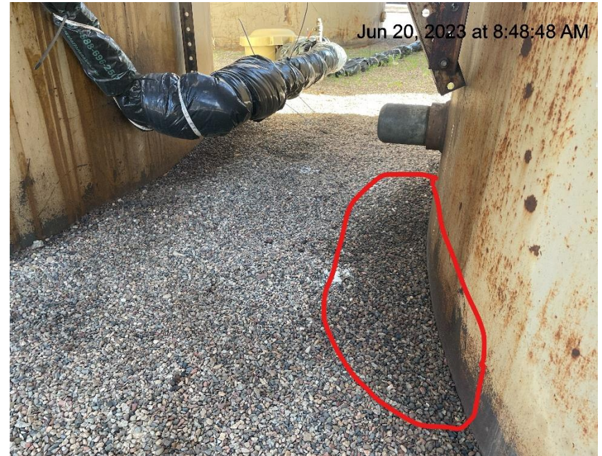
Photo # 991 Stained gravel in secondary containment
