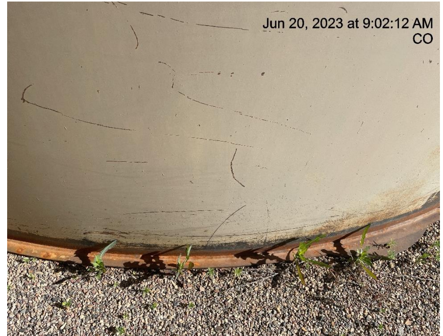
Photo # 1113 Weeds/Undesirable plant species in secondary containment
