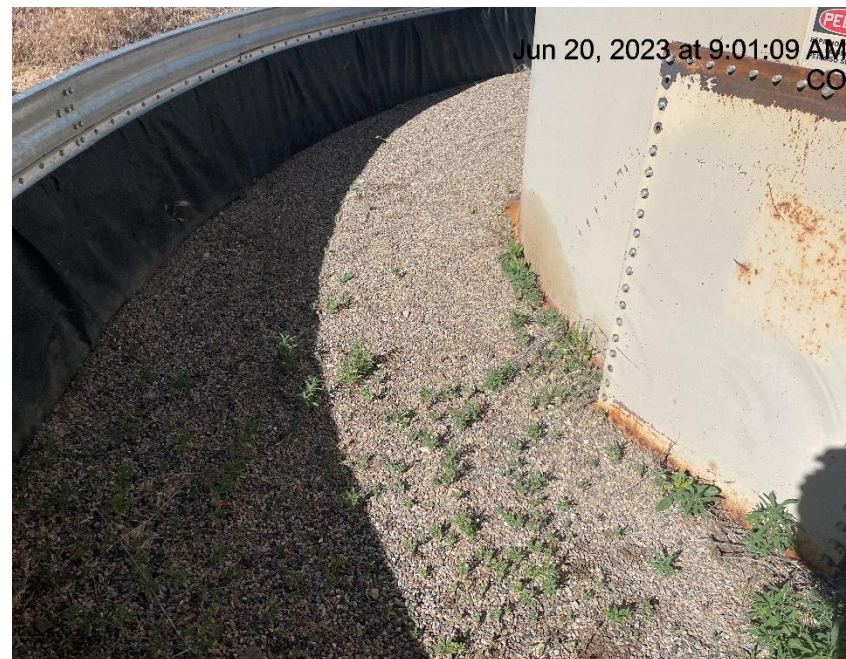
Photo # 1012 Weeds/Undesirable plant species in secondary containment
