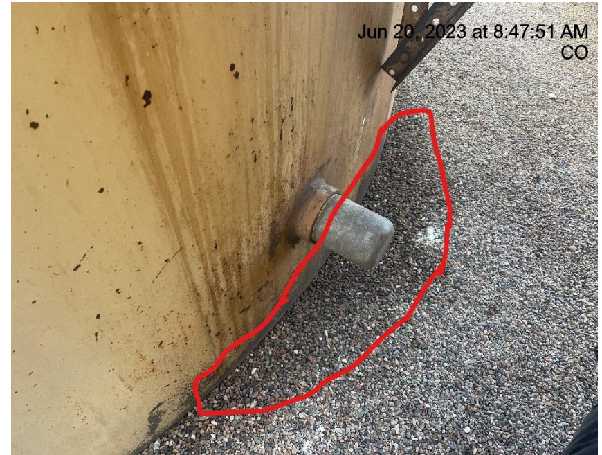
Photo # 987 Stained gravel in secondary containment
