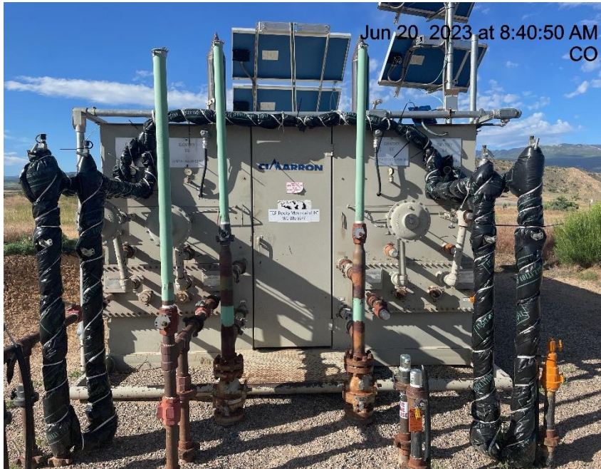
Photo # 978 Meter calibration info not conspicuously posted
