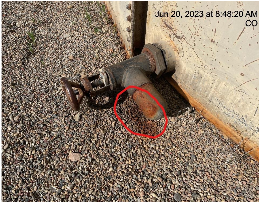
Photo # 990 Stained gravel in secondary containment
