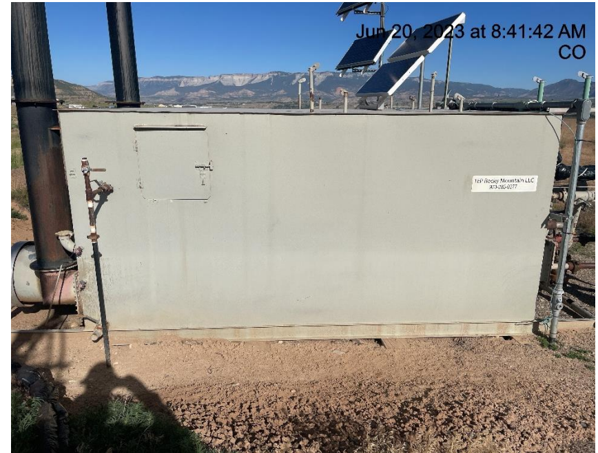
Photo # 981 Meter calibration info not conspicuously posted
