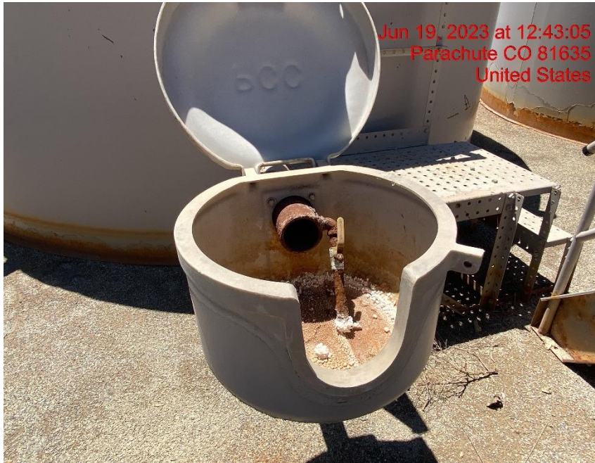
Open-Ended Load Line on Produced Water Tank – Photo #04617
