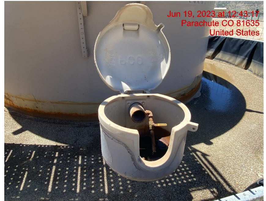
Open-Ended Load Line on Condensate Tank – Photo #04618
