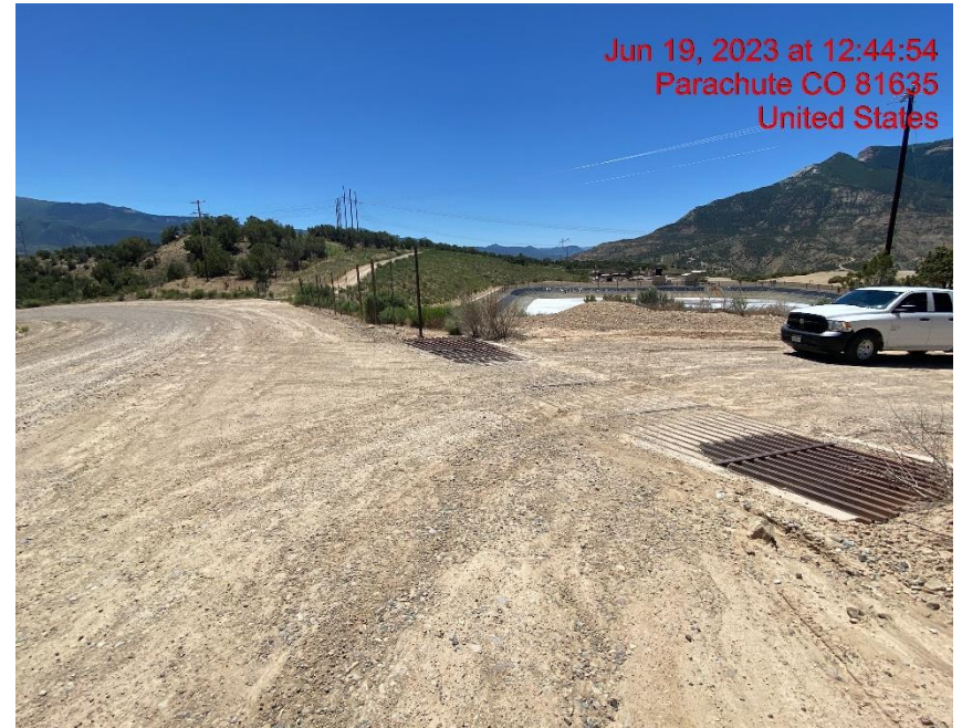
Insufficient Vehicle Tracking BMPs at Location Entrance/Exit – Photo #04625
