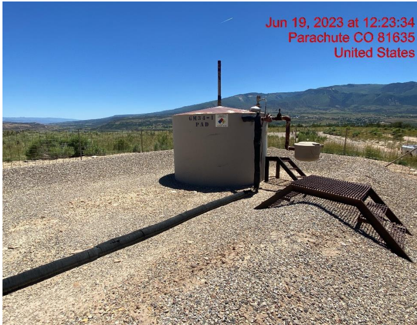
Tank Battery – Photo #04592
