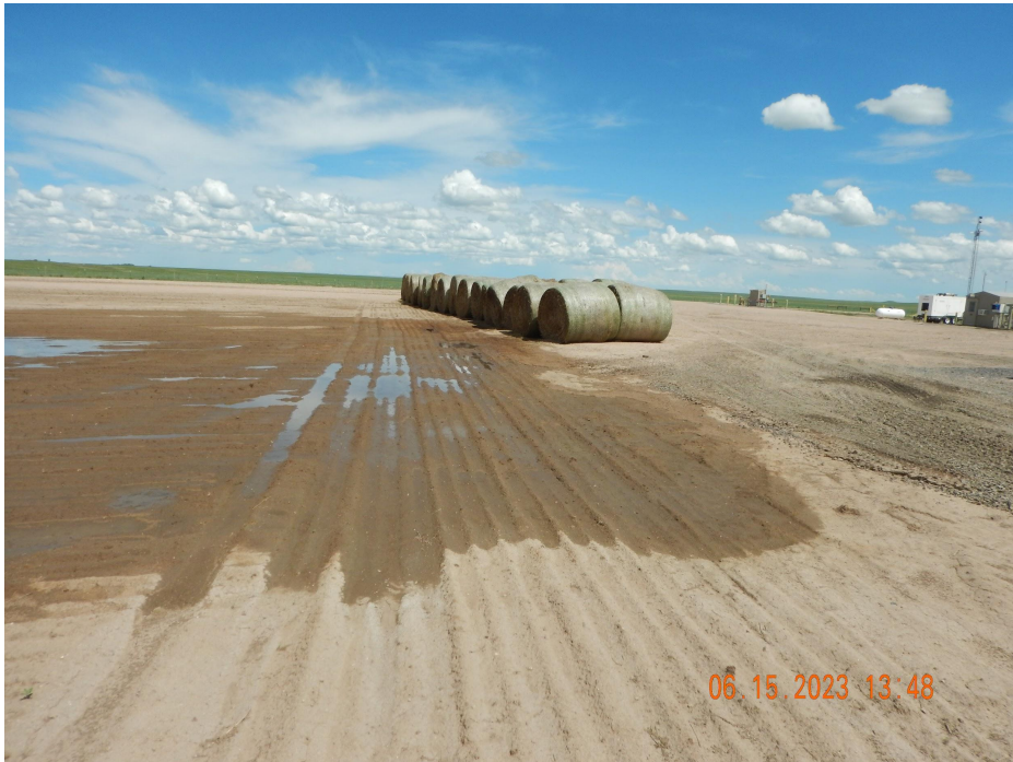
Photo 5. Photo taken from the western interim area, facing East. Photo illustrates straw mulch that appears to be staged for soil stabilization.
