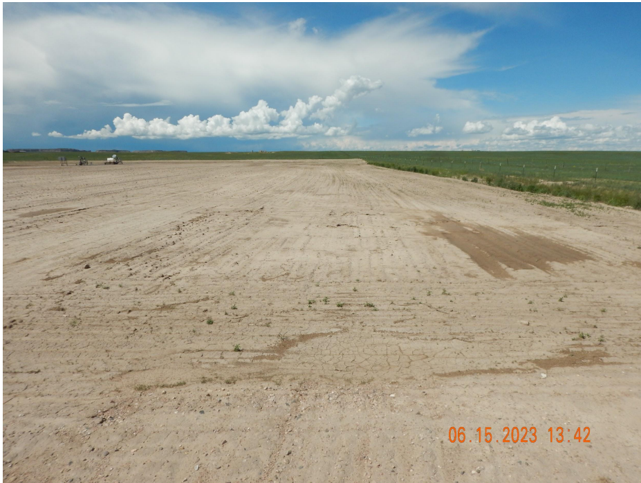
Photo 1. Photo taken from the southeastern location, facing North. Photo illustrates interim reclamation has been performed; however, interim reclamation is not complete due to the lack of soil stabilization. Erosion was evidence and much of the interim reclamation area had no desirable establishment.
