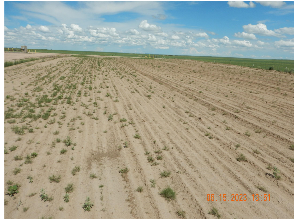
Photo 6. Photo taken from the topsoil stockpile, facing East. Photo illustrates the topsoil stockpile which has been seeded; however, the topsoil stockpile lacks soil stabilization. Some germination of desirable establishment was observed but again lacks soil stabilization.
