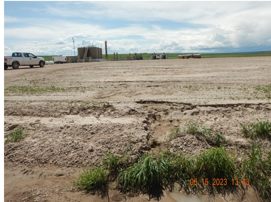
Photo 2. Photo taken from the southeastern location, facing West. Photo illustrates erosion and no soil stabilization.
