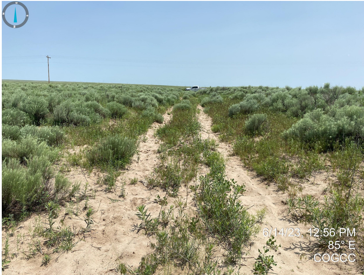
Photo 1. The access road does not appear to have been reclaimed as evidenced by lack of uniform vegetation cover and not contoured to reflect adjacent reference areas.
