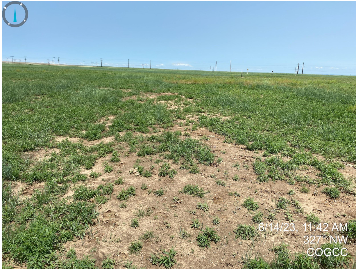
Photo 1. From the start of the former access road. The access road does not appear to be progressing towards Rule 1004 standards with areas of bare soil and undesirable vegetation (e.g. kochia) observed.
