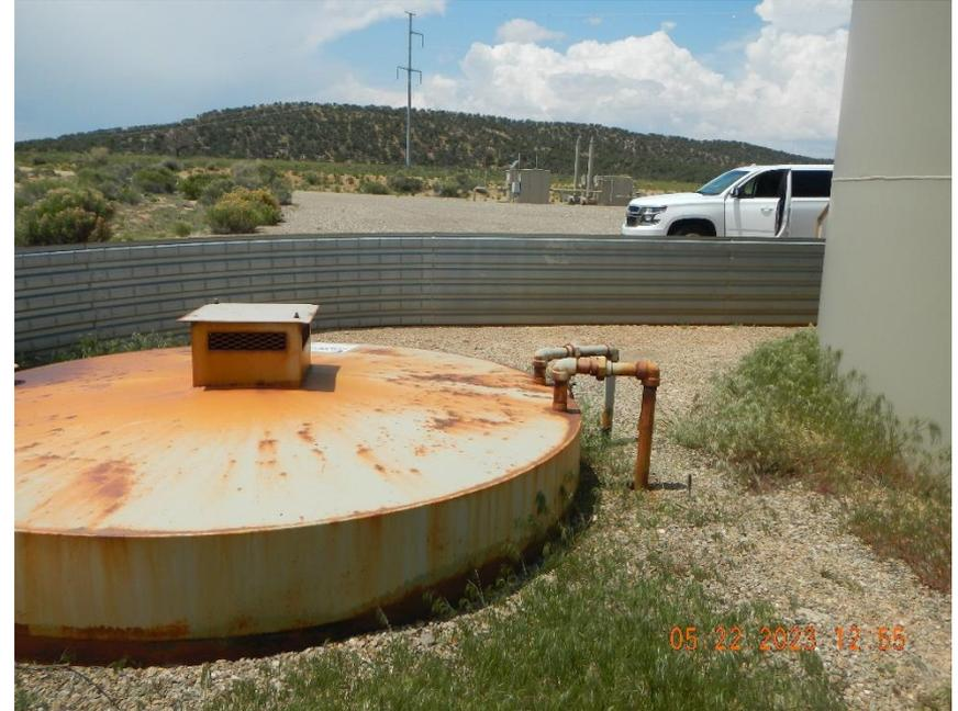
**No label on tank. Rust on tank. Grass growing in berm.**
