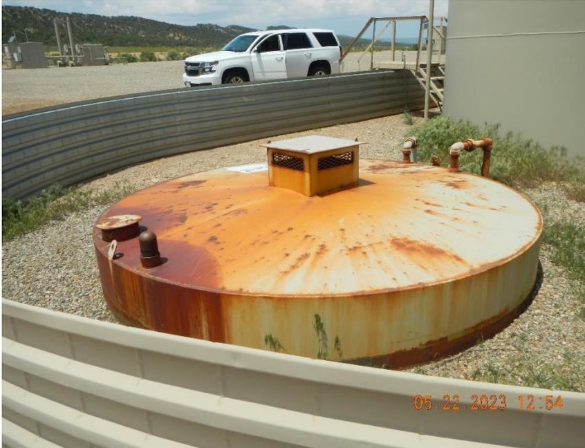
**No label on tank. Rust on tank. Grass growing in berm.**
