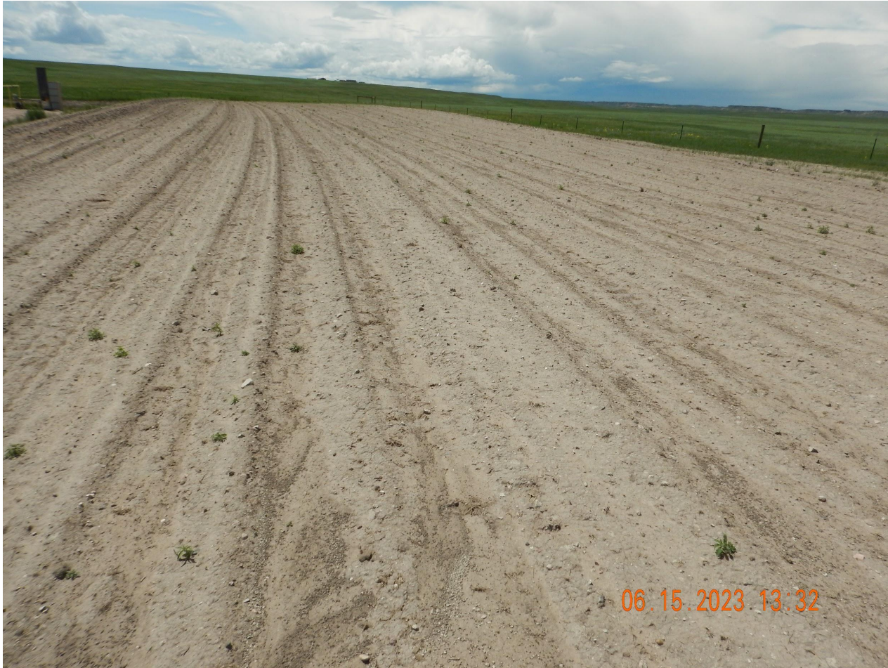
Photo 5. Photo taken from the topsoil stockpile, facing West. Photo illustrates the topsoil stockpile remains unstabilized and no desirable vegetative growth. Weedy annual growth is starting to establish.
