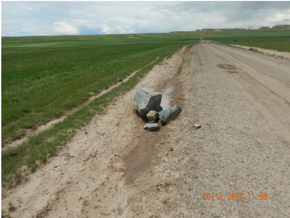
Photo 8. Photo taken from a section of the access road illustrating check dam BMP installation. Operator has not installed the BMP per good engineering practices.
