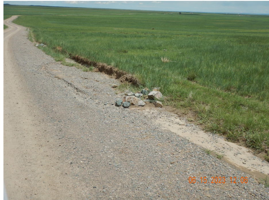
Photo 9. Photo taken from a section of the access road illustrating check dam BMP installation. Operator has not installed the BMP per good engineering practices. Stormwater is going around the BMP, some of which is going into the adjacent pasture.
