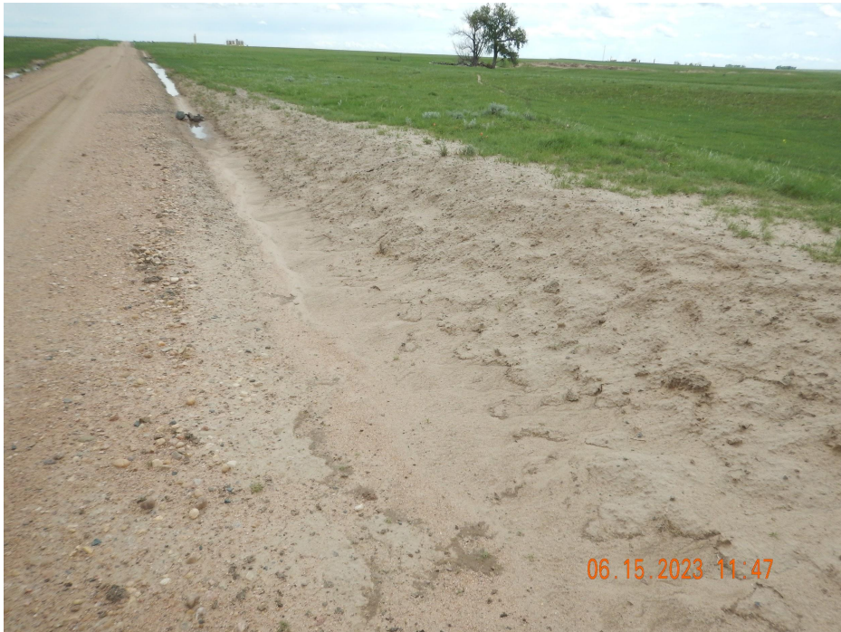
Photo 3. Photo taken east of Geary Creek, facing East. Photo illustrates Upland disturbances along a cut slope of the access road have not been addressed which are related to the original Rule 1002.e. violation and are now eroding into Geary Creek. Refer to Photos 5 & 6.
