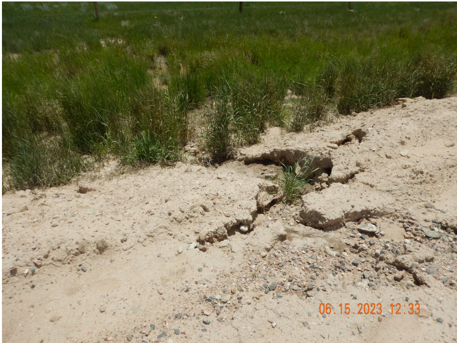
Photo 14. Photo taken from the southern perimeter of location, facing South. Photo illustrates gully erosion in need of repair.
