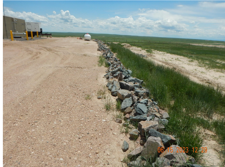
Photo 11. Photo taken from the western perimeter of location, facing South. Photo illustrates Operator has installed a riprap berm along the top of the fill slope.
