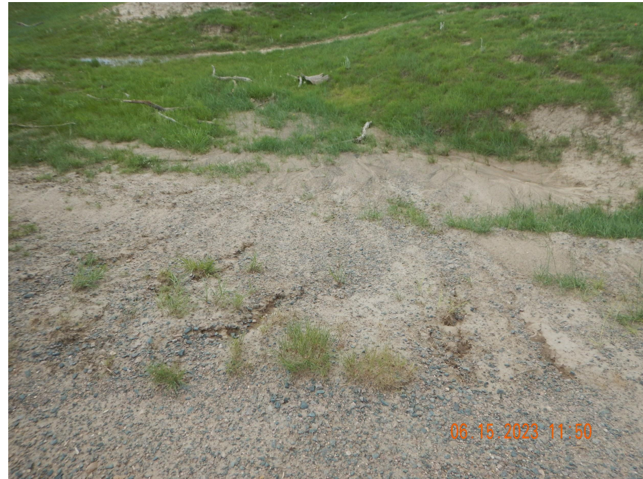
Photo 6. Photo taken east of Geary Creek, facing South. Photo illustrates sediment laden stormwater discharging into Geary Creek without any stormwater BMPs.
