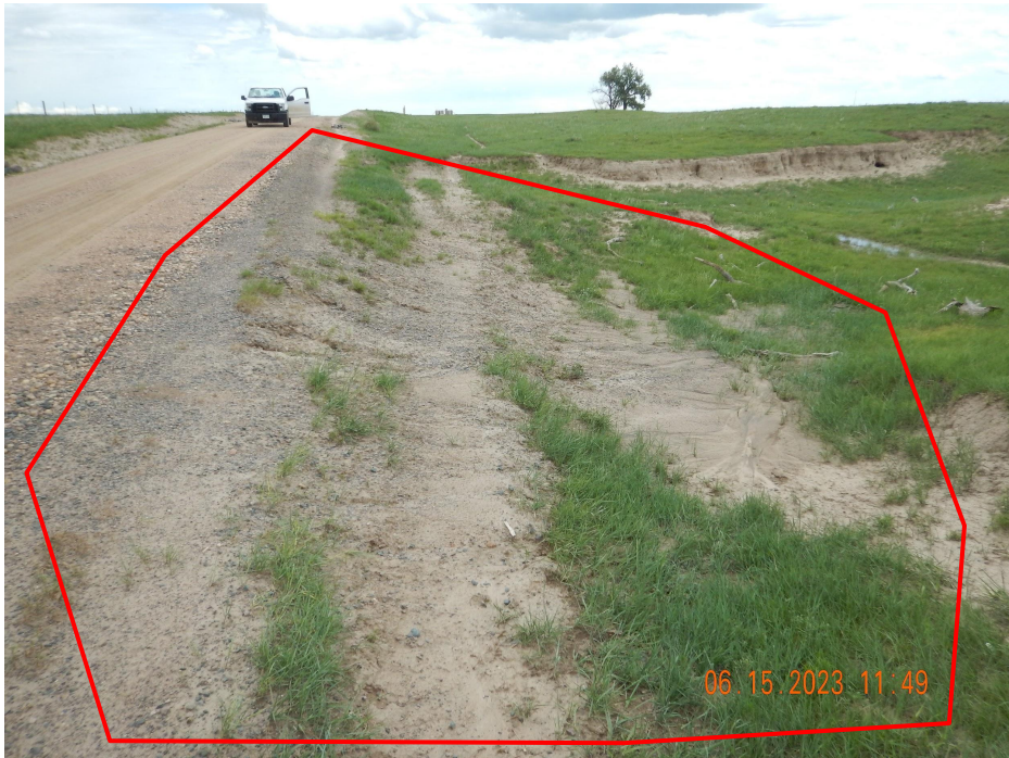
Photo 5. Photo taken from Geary Creek, facing East. Photo illustrates sediment laden stormwater discharging into Geary Creek from Upland disturbances without any stormwater BMPs.
