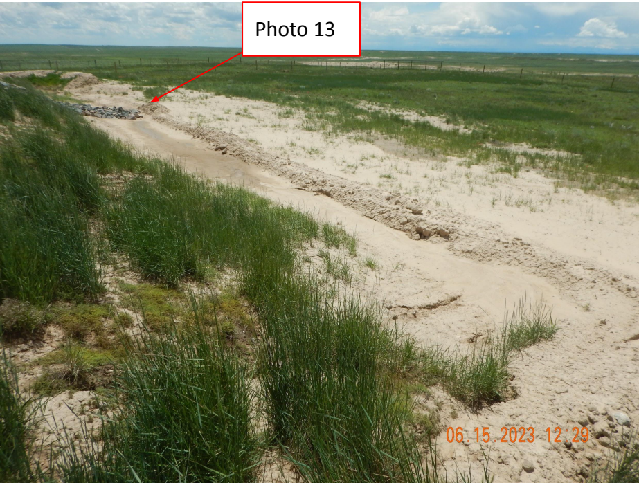
Photo 12. Photo illustrates a berm BMP installed along the toe of the fill slope, facing South. Berm BMP has not been installed per good engineering practices.
