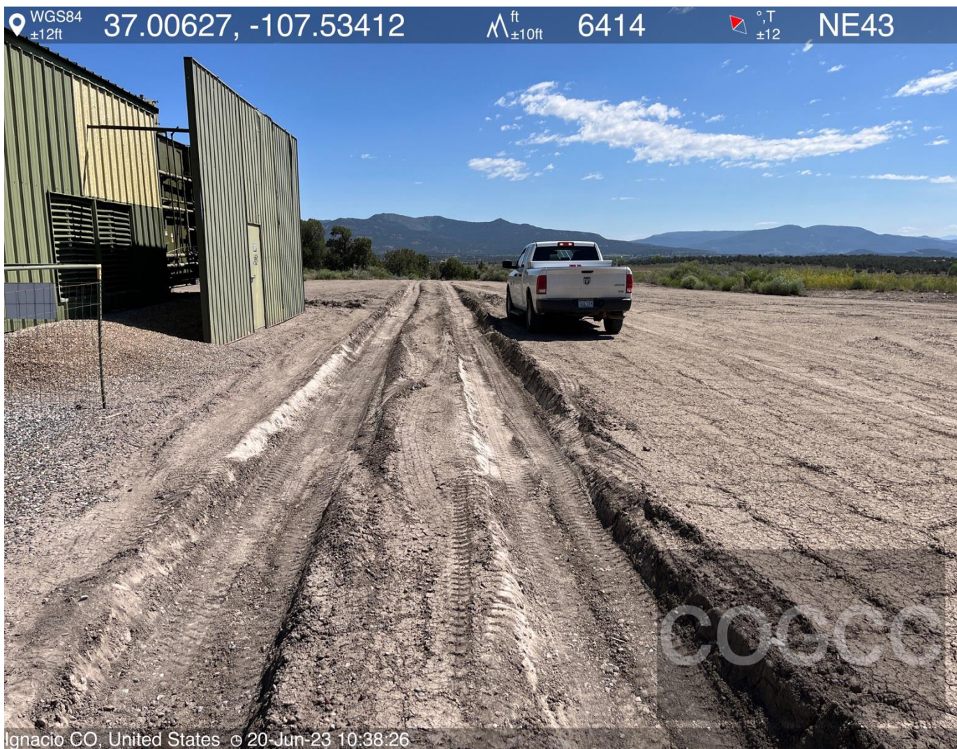
Photo #3 View of rutting on well location.
