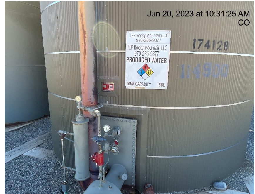
Photo # 1168 Tank label missing required information
