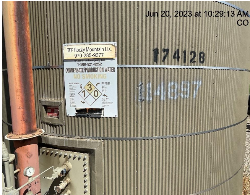
Photo # 1158 Tank label missing required information
