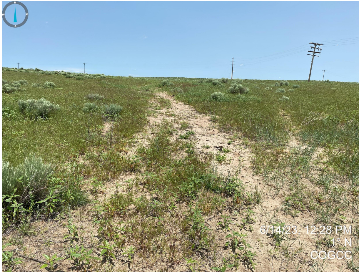
Photo 2. Access road leading to the former well location does not appear to have been reclaimed. Colorado List C Noxious Weed (cheatgrass) observed to be growing throughout the former access roads and well location.
