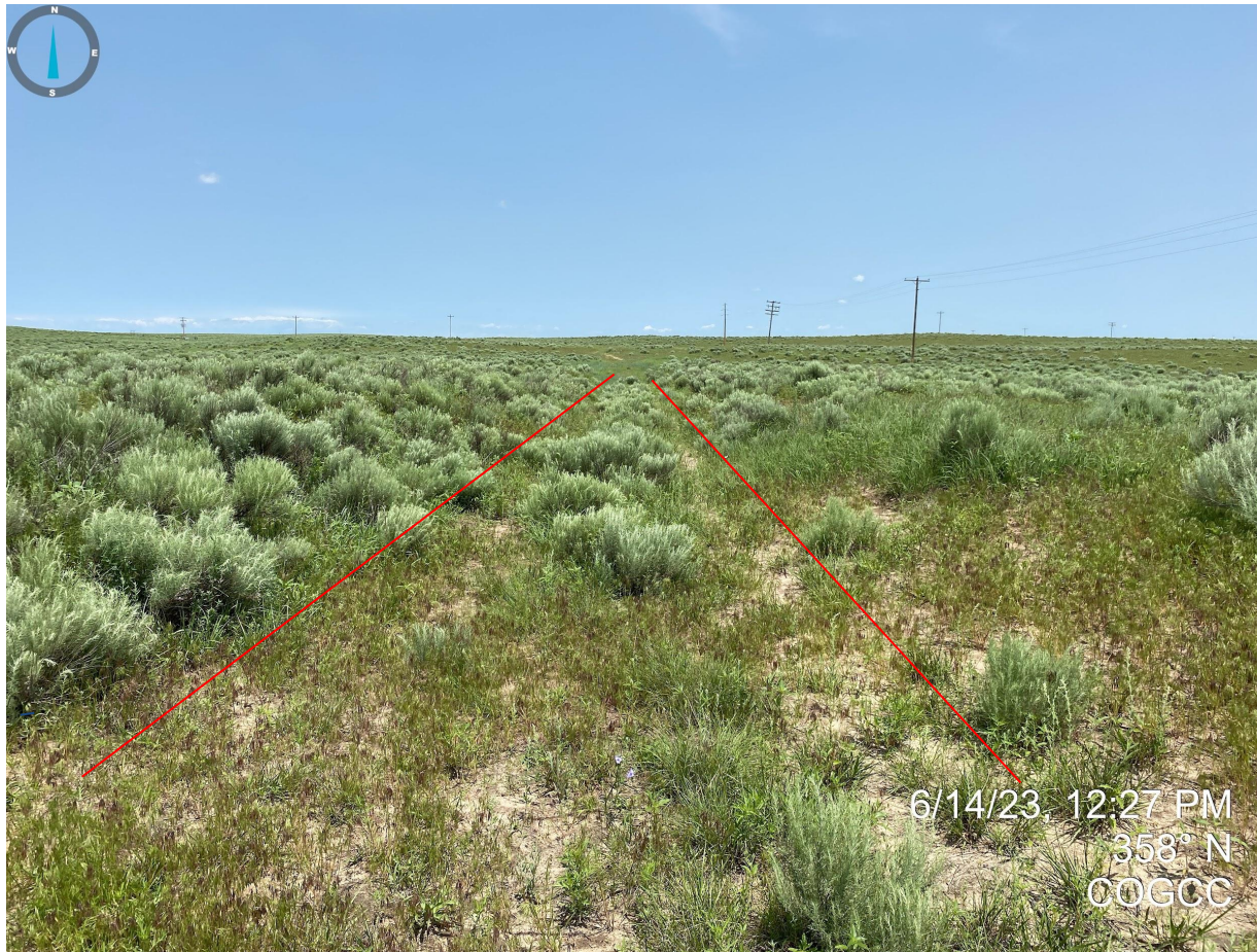
Photo 1. Facing north at the start of the access road. The access road does not appear to have been reclaimed as contouring issues were observed. Banks on each side of the access road were approximately 2-3' higher than the access road.
