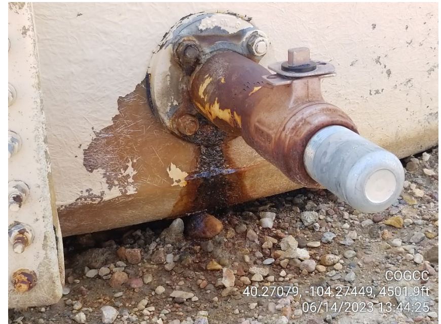
Photo 8 – Back Drain Leaking
