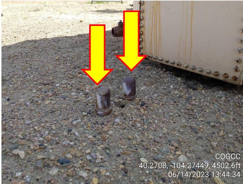
Photo 9 – Unmarked Risers
