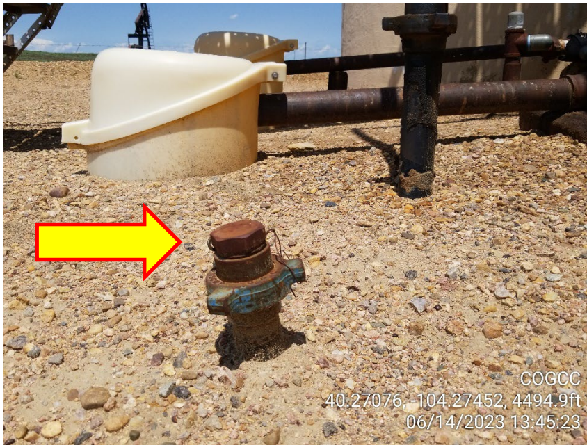
Photo 13 – Unmarked Riser
