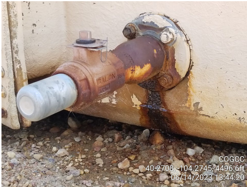
Photo 7 – Back Drain Leaking
