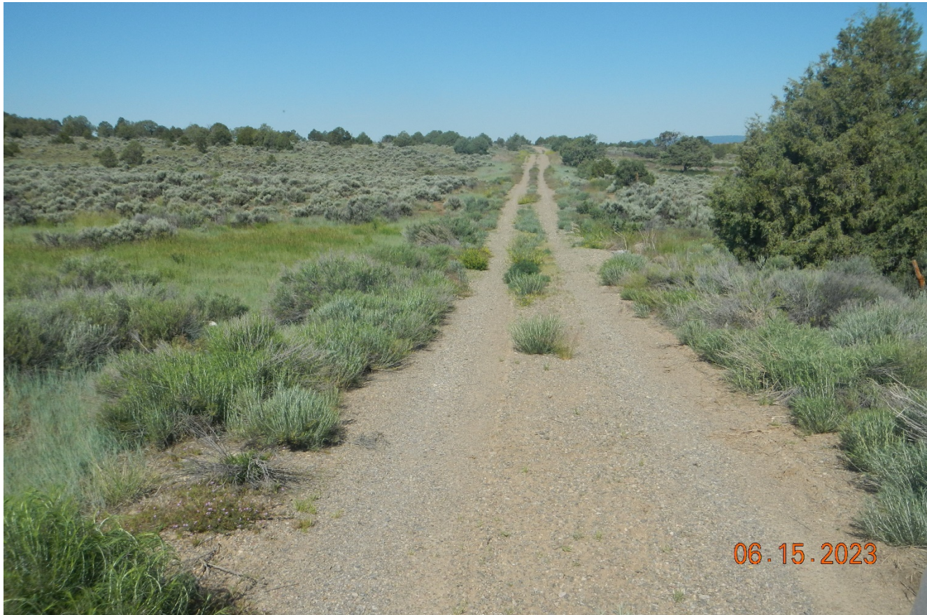
Photo 1. Facing west along the access road.
