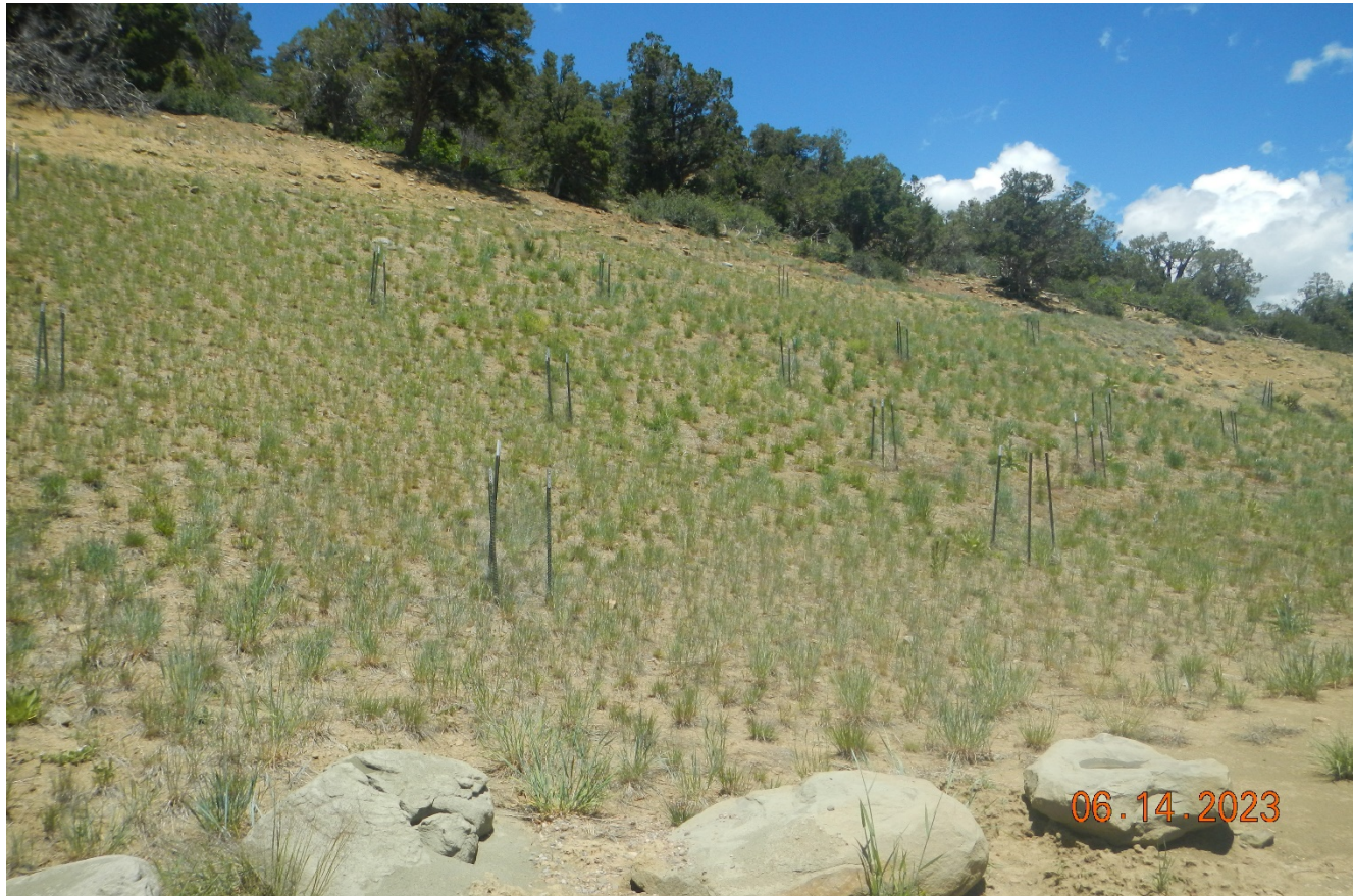
Photo 2. Facing toward the cut slope which appears stabilized with vegetation.
