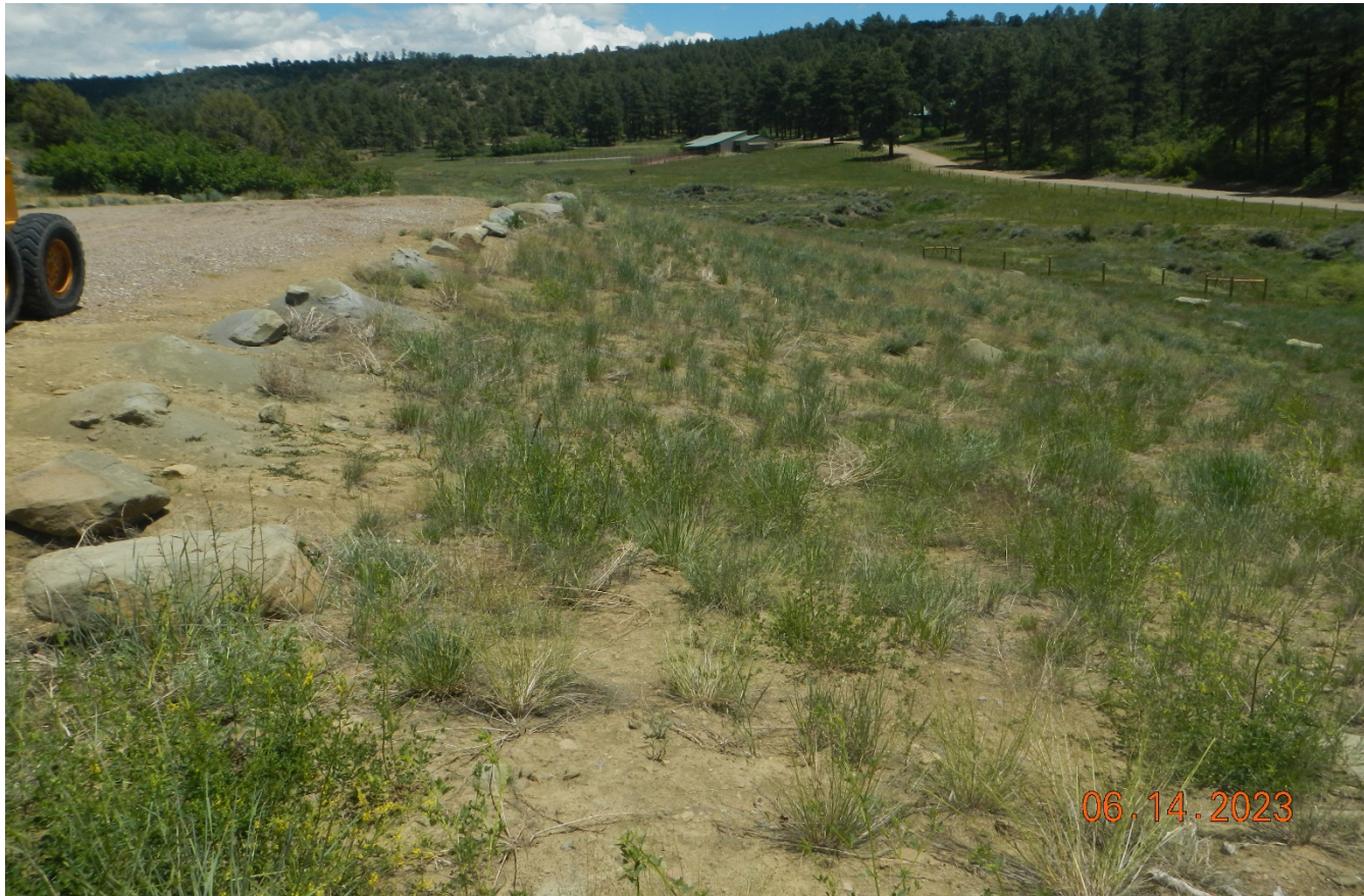
Photo 5. Facing toward the fill slope.
