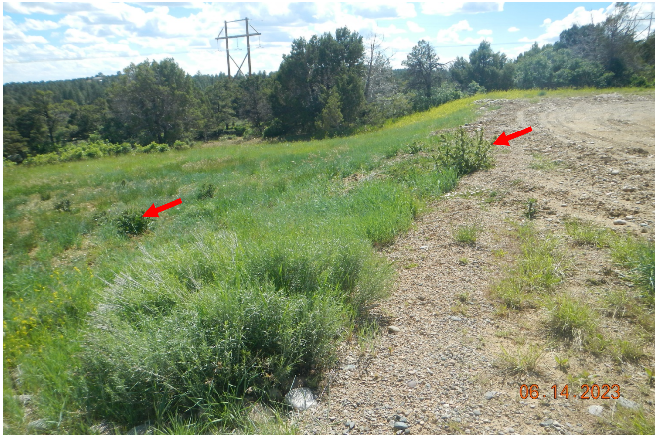
Photo 2. Facing toward the south fill slope which appears stabilized with vegetation. There are noxious weeds in this area that need to be controlled. Red arrow points to Musk thistle.
